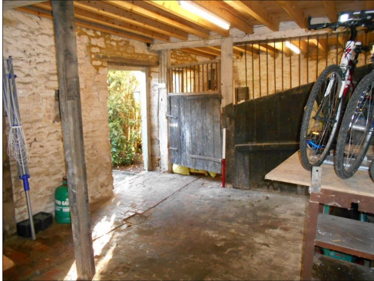
Fig 9: The interior, western part, looking south-west, showing the common-brick floor, with travis and door in background; scale 1m
