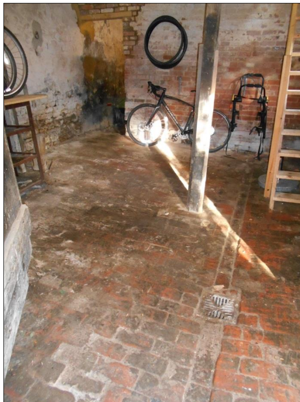
Fig 10: Interior, western part, looking north-east. Note the floor of common bricks laid on-bed, with simple integral drainage gully
