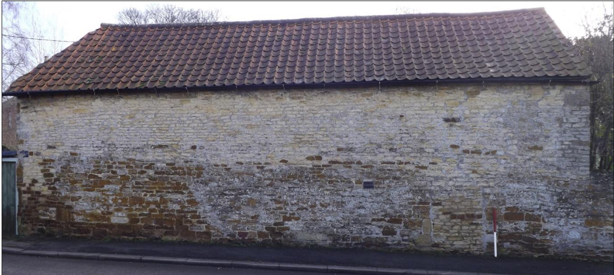
Fig 6: View south across Draughton Road. This shows clearly the two-phase north wall built off a former boundary wall with blocked pedestrian doorway; scale 1m
