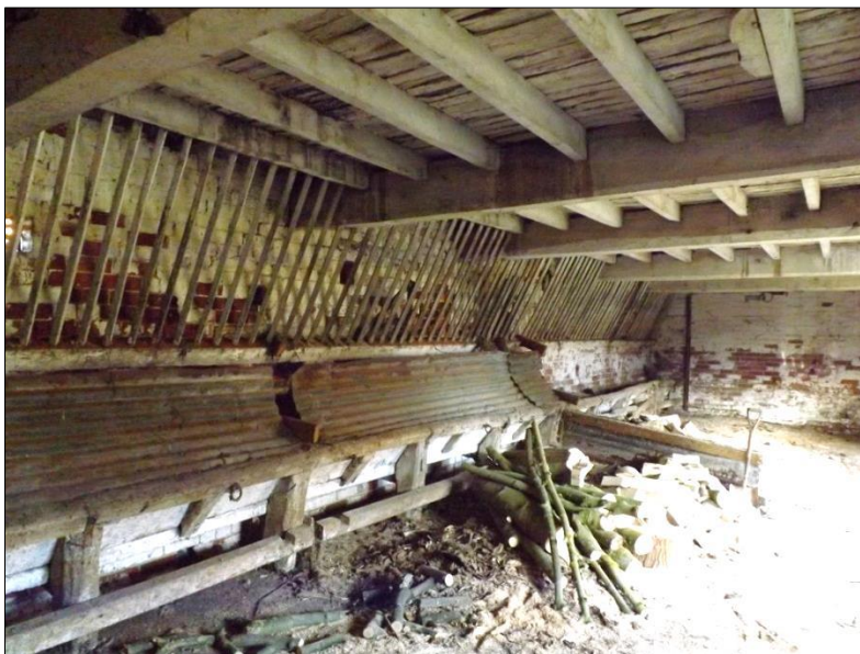
Fig 11: for comparison: timber manger and hayrack at a stable in Warwickshire
