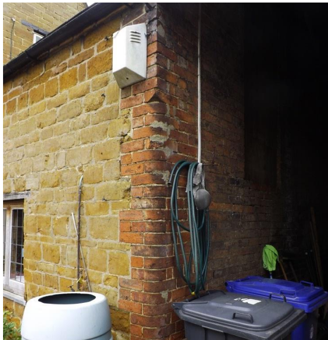
Fig 12 South-east corner of Phase Two showing bull-nose bricks and neat quoin joint
