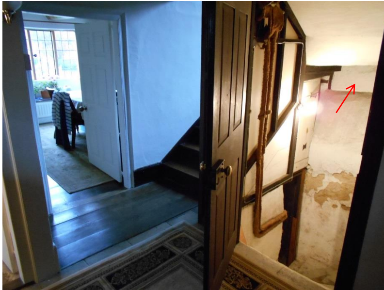
Fig 14: Door to cellar in north wall of G3, the rear hall, looking north-west; the blocked cellar window reveal is arrowed
