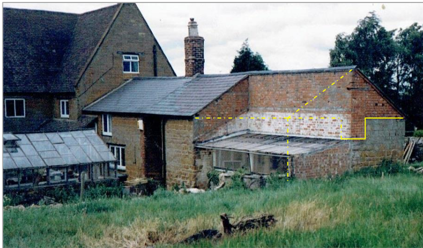
Fig 7: The form (in yellow) of the phase 3 stone outbuildings prior to a) partial brick rebuild with two phases of lean-to greenhouse and b) remodelling to form the current garage
