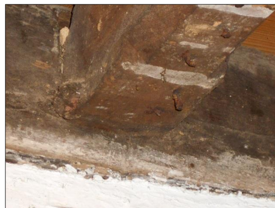
Fig 6: Stopped chamfers on the ceiling joists of the kitchen (former parlour).
