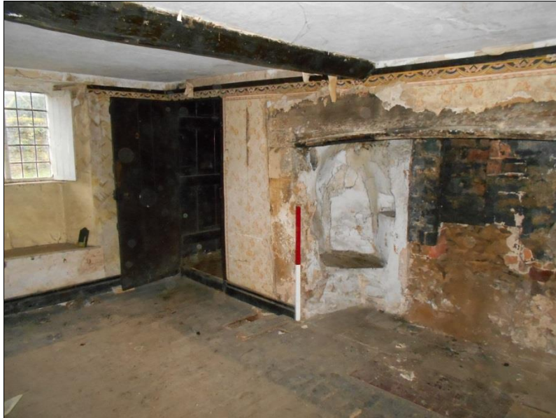
Fig 2: The western room (hall), fully cleared, looking south-west towards the front door; scale 1m. Under the timber floor was a void of some 300mm, and beneath that, a skim of concrete over the natural ironstone.
