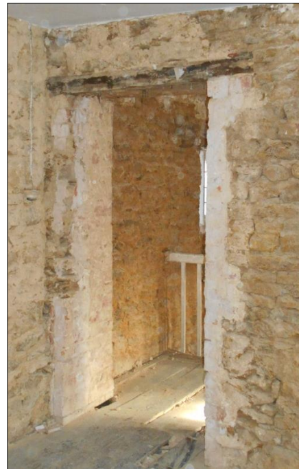
Fig 13: brick doorway alteration between bedrooms
