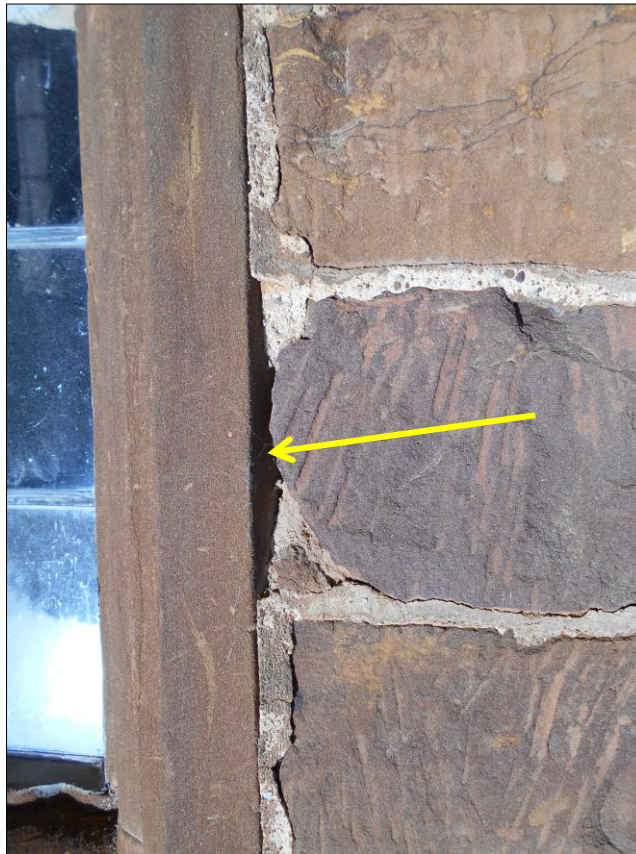
Fig 15: A built-in face to a former mullion, reused as a jamb (south-wall, east room exterior)
