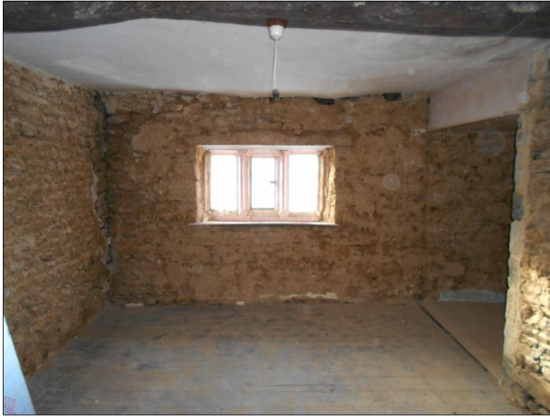
Fig 11: The western bedroom, pared back to the stonework, looking south.
