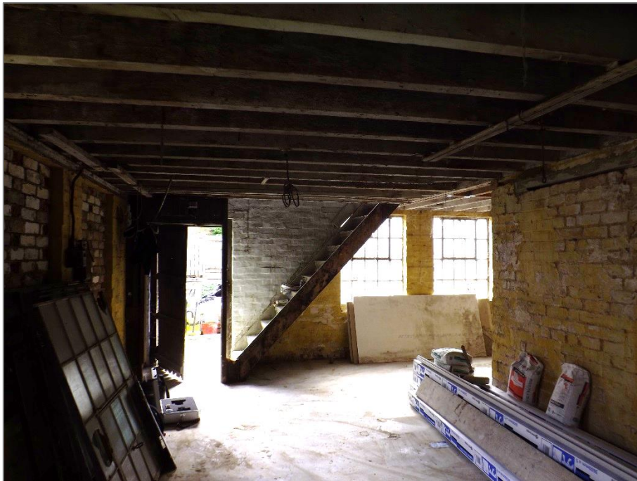
Fig 8: Ground floor, looking east
