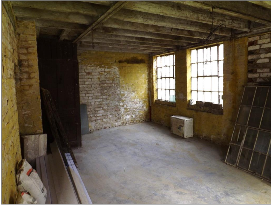
Fig 9: Ground floor, looking north-west
