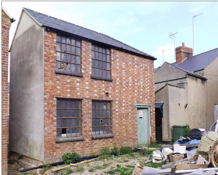
Fig 5: East elevation, looking north
