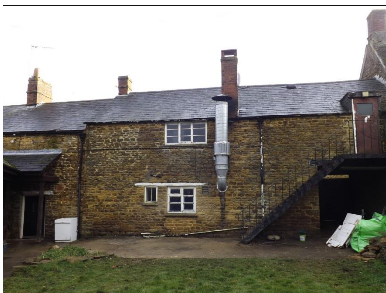
Fig 12 : The rear elevation of the service range; the main block is covered by 20 th -century accretions at the north end
