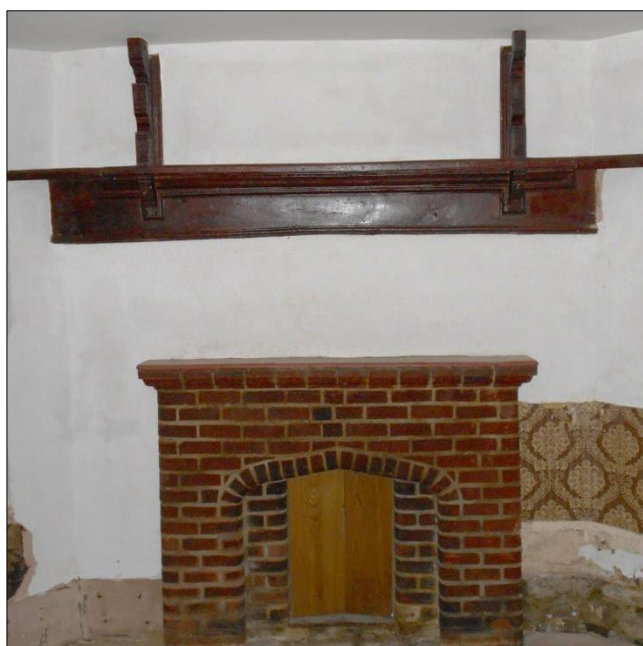
Fig 16: G6 – Small corner fireplace and oak spit-rack above.
