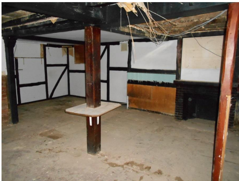
Fig 13: The main pub interior; all internal walls taken out to improve circulation and finished with inappropriate decor
