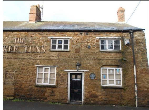
Fig 7: The old core of the building (1690)
