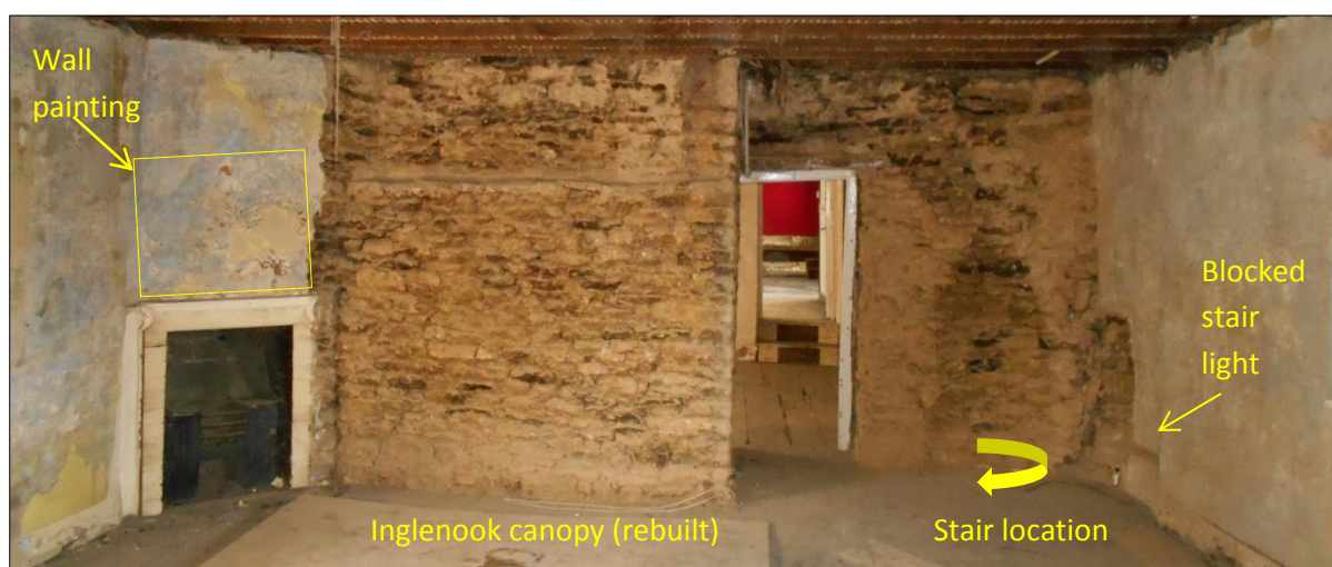
Fig 19: the south side of room F3; fireplace and wall-painting to left, stair to right
