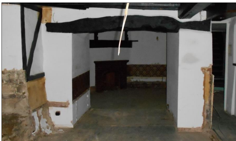
Fig 14: The knocked-through inglenook from the front (G5). The stair one stood to the right. Note the spit-rack (see below), glimpsed in G6 beyond
