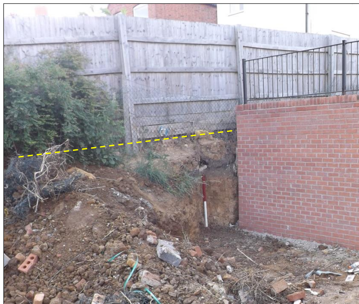
Fig 3: The earlier terrace being uncovered by the removal of builders' rubble; scale 1m. The dashed line shows the old ground surface cut back to build the car park wall.
