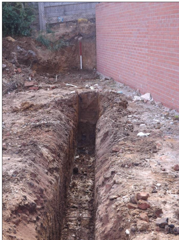
Fig 4: View east along the southern side of the new house foundations, showing the extent of truncation in the existing terracing behind; scale 1m
