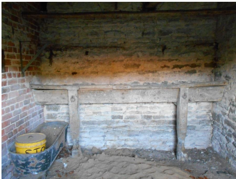
Fig 22: The stable with surviving manger looking west; the hayrack has disintegrated
