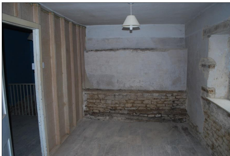
Fig 15: Room F2, and F1 through the doorway. This plain room is formed with flimsy partitions, latterly papered over.
