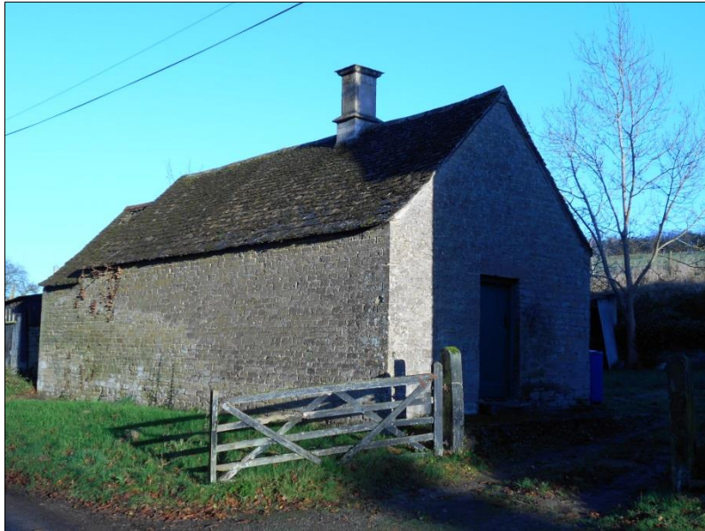
Fig 18: The outbuildings, viewed from Causin Way
