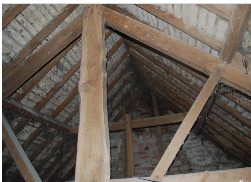
Fig 17: The roof truss and collar, looking west
