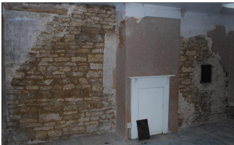
Fig 16: Room F3, western gable, showing the old roof line and the blocked window behind the inserted chimney and fireplace.
