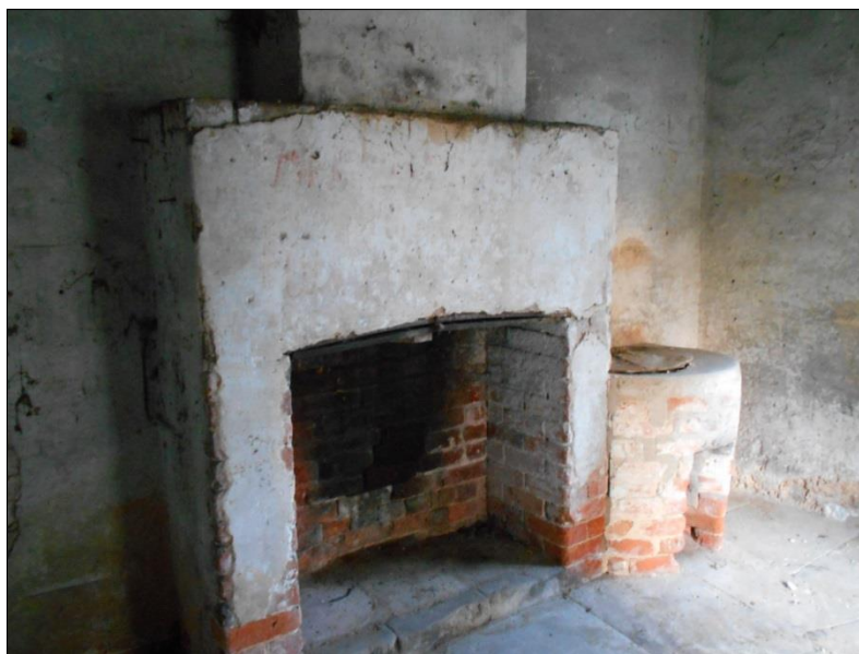
Fig 20: The wash-house with its brick fireplace and copper
