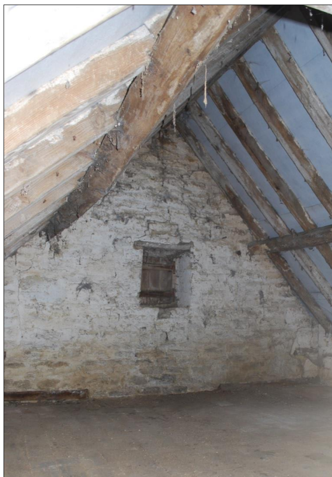
Fig 13: Store room above bread oven, looking east
