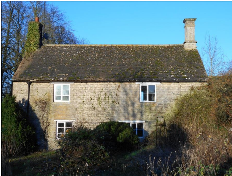
Fig 8: the south-facing elevation of the cottage.
