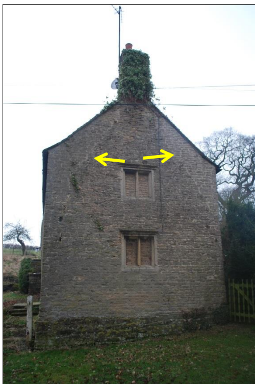
Fig 5: The road-side (west-facing) gable, with blocked windows; note the early gable-lines (arrowed)
