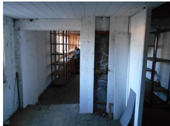
Fig 11: Boarded-out chimney breast rising through F1, looking south into F beyond
