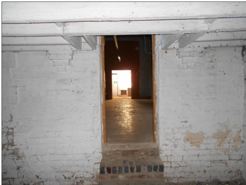
Fig 9: The inserted north doorway through an older, wider opening from G1, looking north into G2. Note the level change and the brick corbels and trimmed joists above which facilitated the doorway-height
