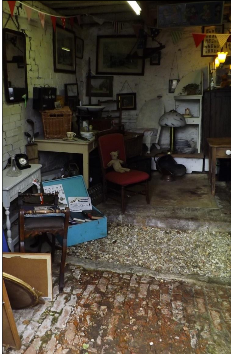
Fig 8: The stable interior showing brick flooring, gravel-filled drainage channel and raised stall area. Looking north.
