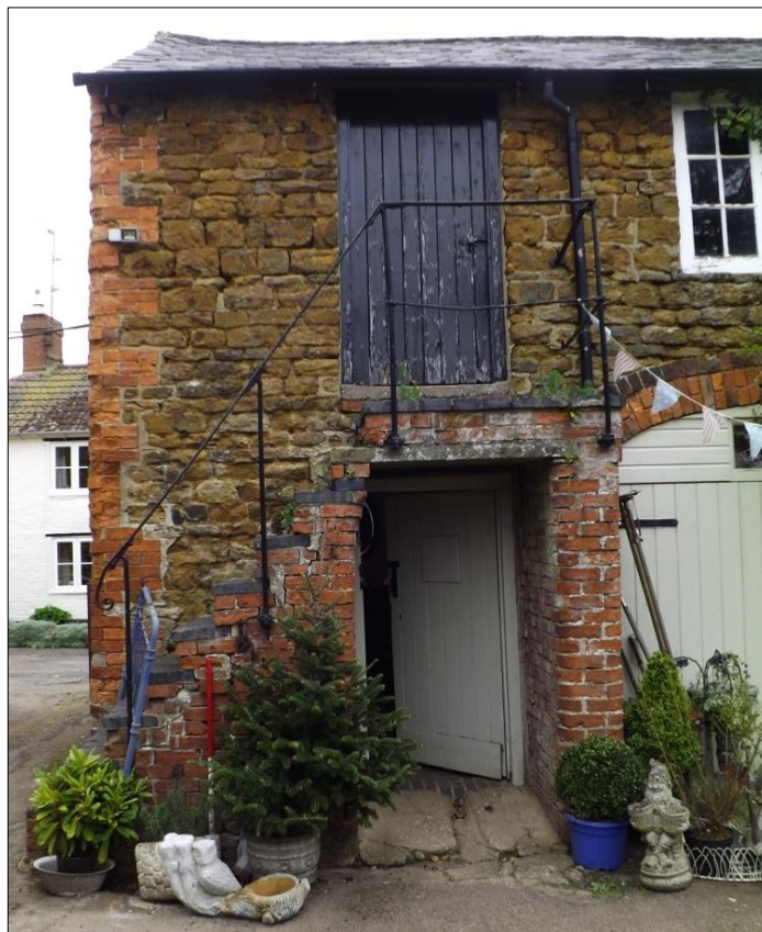
Fig 9: The external stairs, looking north; 1m scale.
