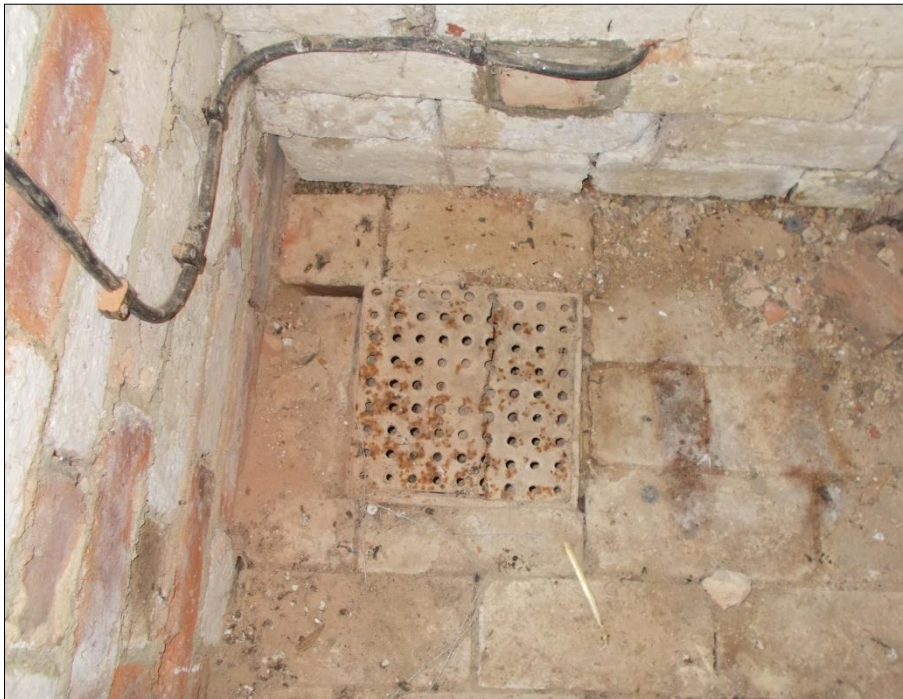
Fig 8: The floor and drain with cast iron cover.
