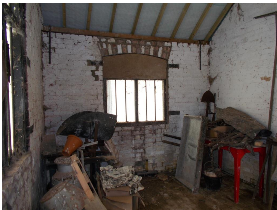
Fig 6: The window in the south wall, looking south.
