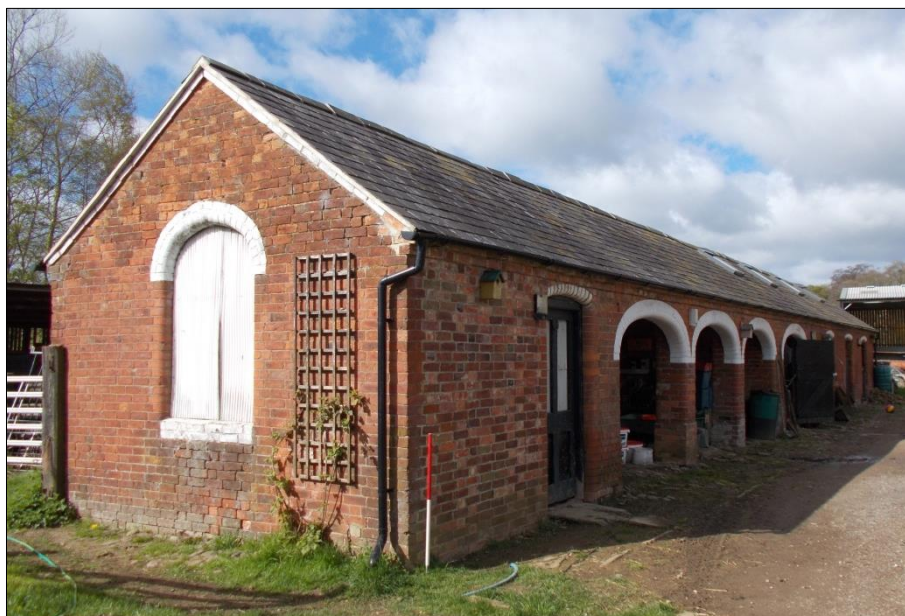
Fig 2: The brick range containing the former meat larder which is located in the foreground behind the arched window in the gable wall. Looking south-west; 1m scale.
