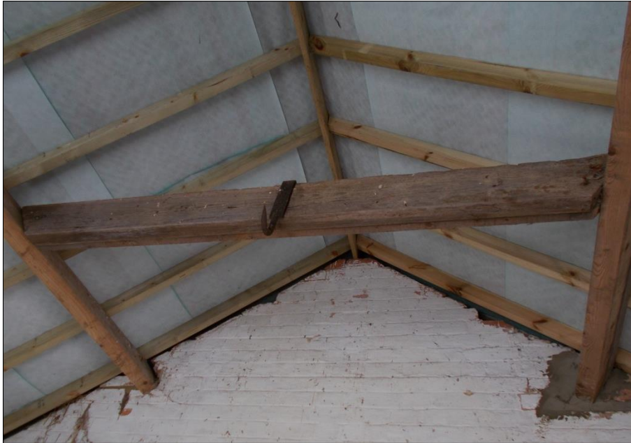
Fig 7: The meat hook on the west collar, looking south-west.
