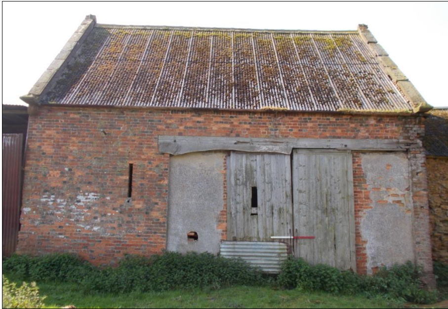
Fig 5: The north elevation of the field barn, looking south; 1m scale.
