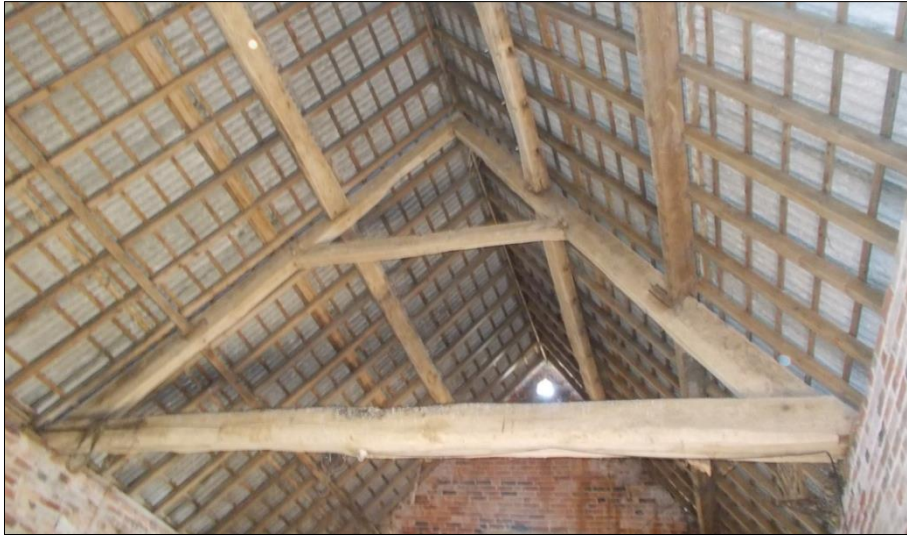
Fig 10: The roof of the field barn, looking east.
