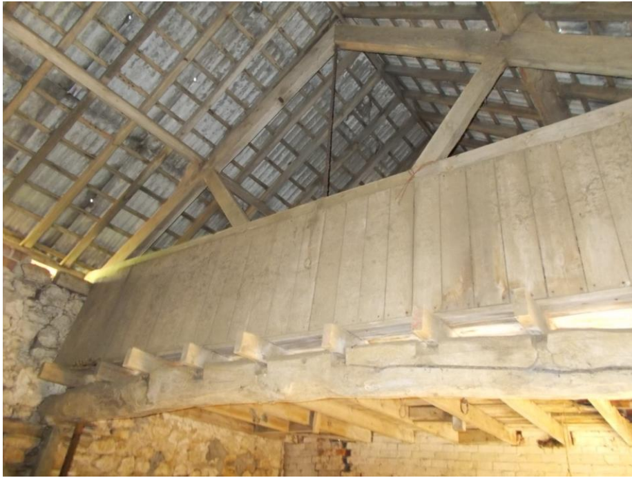
Fig 14: The roof truss and hay loft rail, looking north-east.
