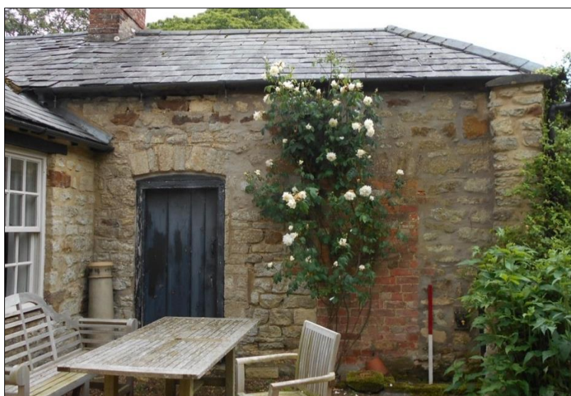
Fig 5: The two doors to the former implement shed (right, blocked in brick), and the produce store (left, blocked on the inside); scale 1m
