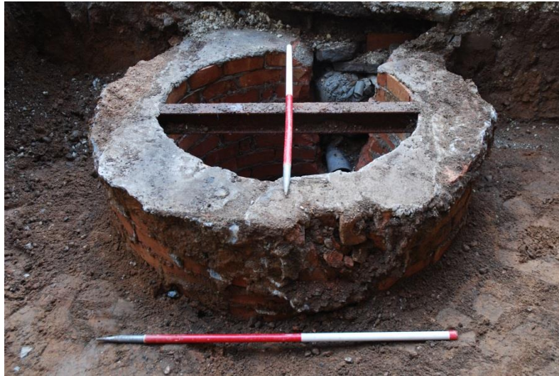
Fig 4: The well, capping removed, showing the rebuilt uppermost courses, RSJ and overflow pipe, looking south-west; scales 1m
