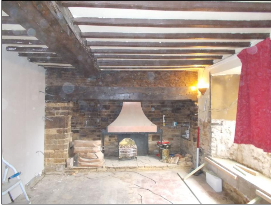
Fig 8: The inglenook looking west; 1m scale.
