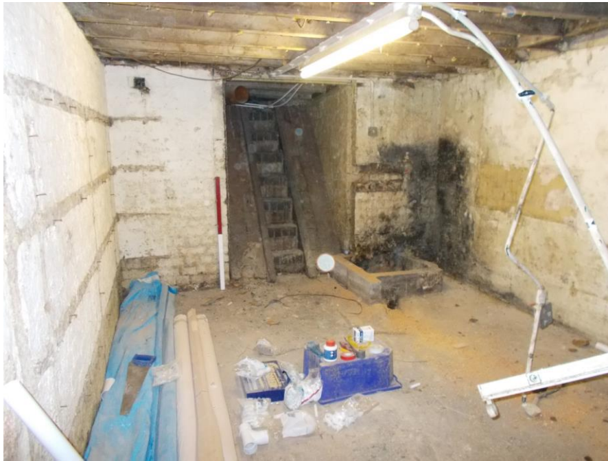
Fig 13: The nineteenth-century cellar, looking south towards beer barrel chute. 1m scale.
