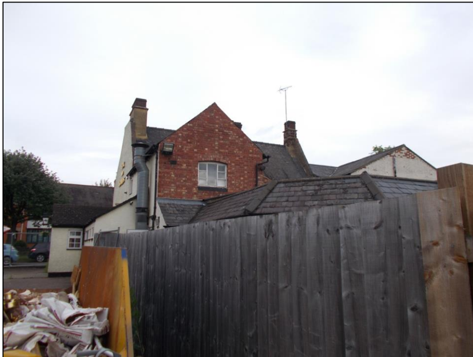
Fig 12: The nineteenth-century additions against the south side of the original building, looking north-east.
