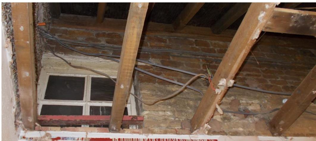
Fig 11: Original west wall of the eighteenth-century building showing banding at first floor level. Note also blocked window placed to light the original stairwell. Looking east (and upward).
