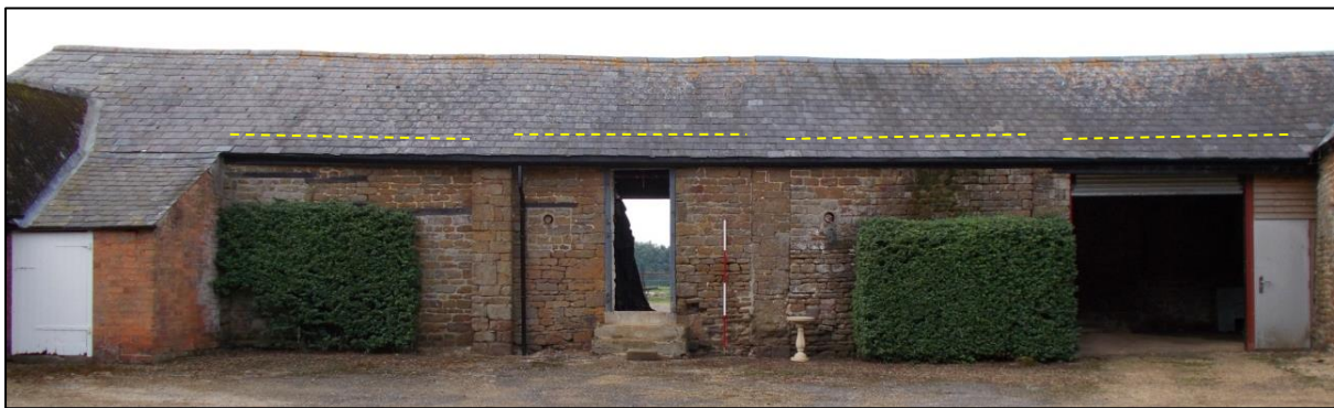
Fig 15: The east elevation of the west range, looking west, infilled bays marked; 2m scale.
