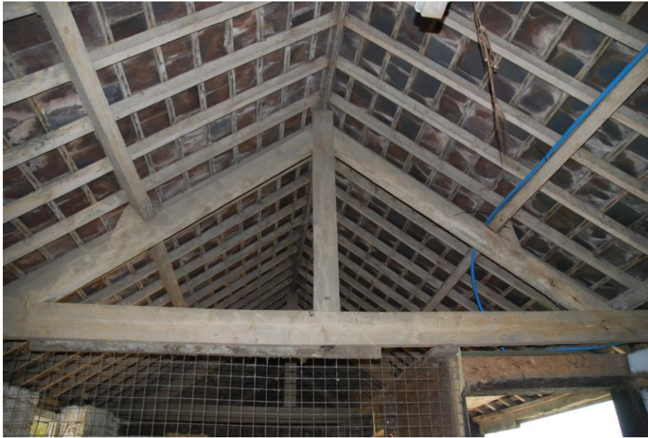
Fig 16: The roof trusses of the west range, looking south.
