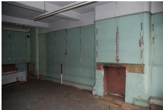
Fig 93: Room EF07, looking north-west; scale 1m
