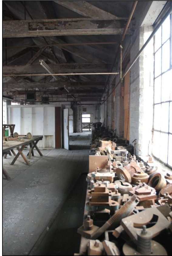
Fig 62: ES29 looking east. Stacked press fittings.
