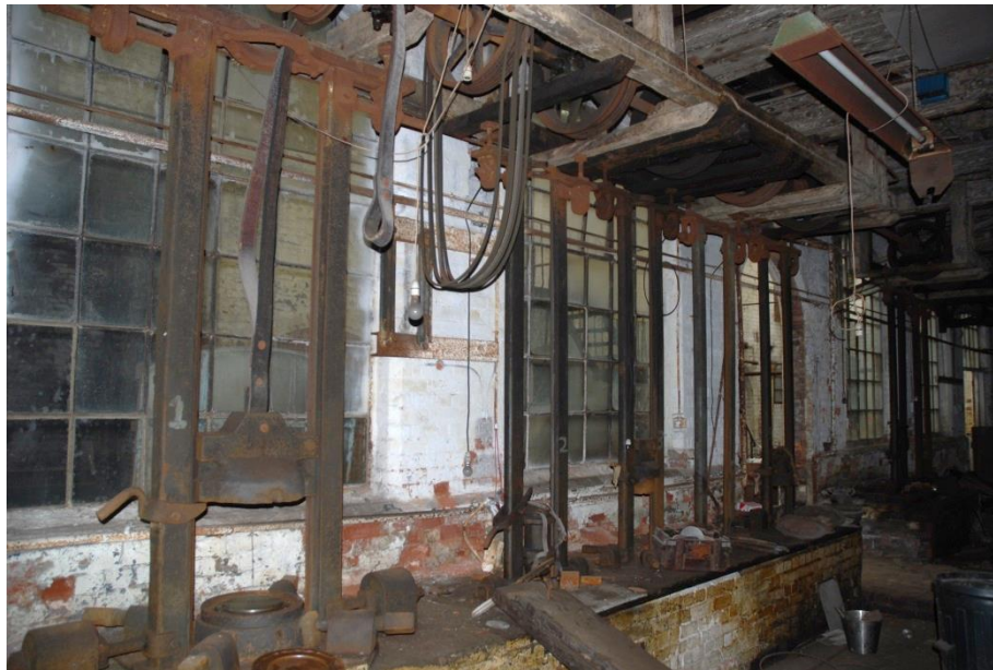
Fig 47: View showing the bench, surviving battery of presses, and timber cradle with driven wheels on a spindle or shaft. The nearest press (also shown in the figure below) has been left with a manual pull-belt for individual stamps for engaging the power, carefully and slowly.
