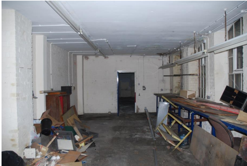
Fig 100: Room EG19 looking west. There was formerly probably an annealing hearth on the left against the wall
