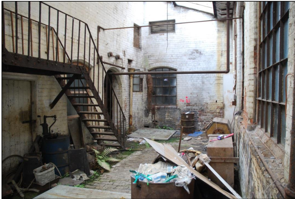
Fig 77: The covered yard EG29, looking west towards the rebuilt gas-engine house. Note the mains gas pipe crossing the yard from right to left. This was traced back all the way to the frontage.
