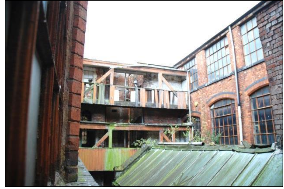
Fig 27: View west over Polishing shop of the two-floor timber link walkways between the two principal workshop ranges. EF59 and ES39 to right
