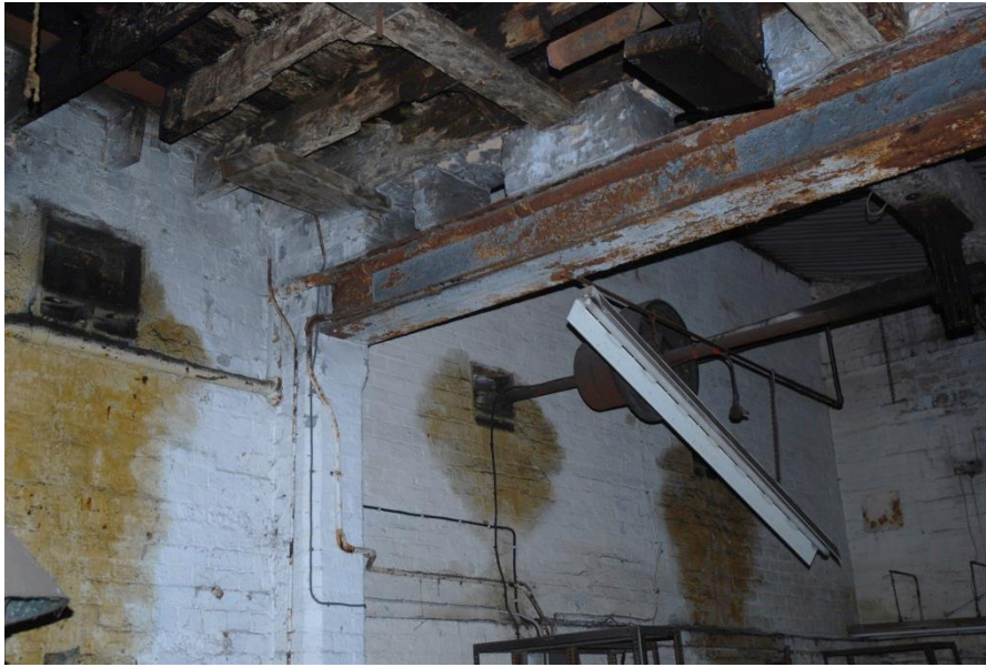
Fig 51: View around the western end of EG49 looking north-west into what was originally the Blacksmith's Shop until at least c1897. The bearing-ends and grease-marks on the wall of three former driven shafts can be seen (with one left in situ). Above the RSJ in the ceiling can be seen a series of slots, through which the drive and relay-belts passed unhindered.
