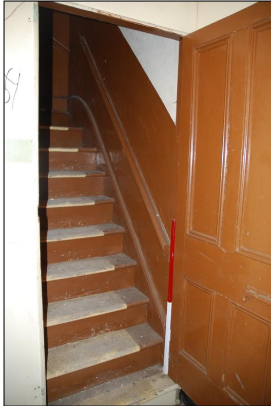
Fig 95: Staircase from Room EF04, is part of the Victorian/Edwardian ensemble and the door matches the one in EF03; scale 1m.
