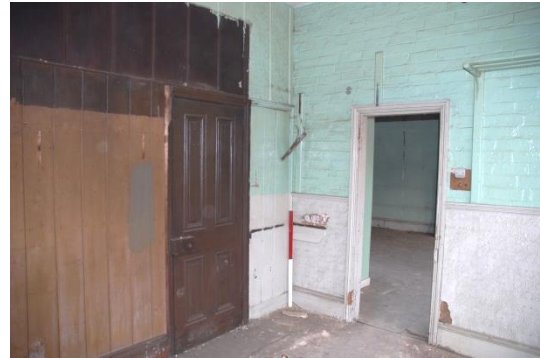
Fig 92: Room EF03 view of panelling and anaglypta wall-covering; scale 1m
