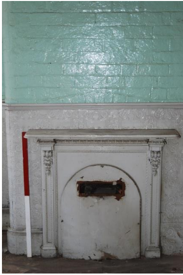
Fig 91: Room EF03 fireplace; scale 1m
