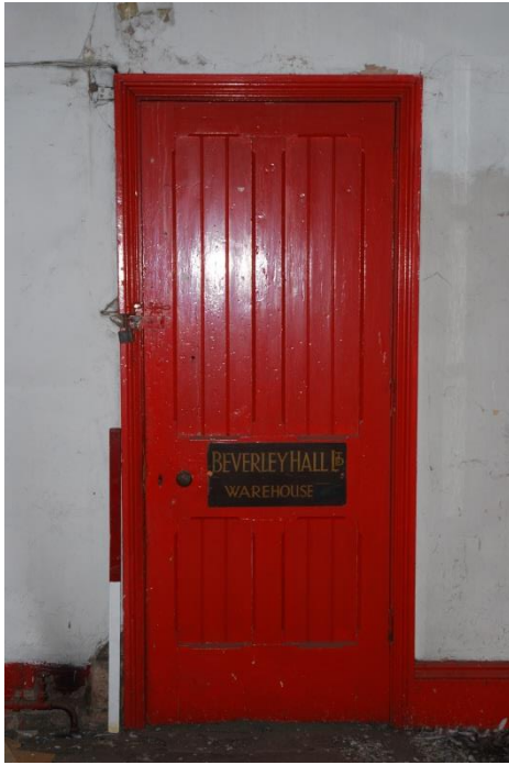
Fig19: The door to EF64, the Beverley Hall Ltd warehouse; scale 1m
