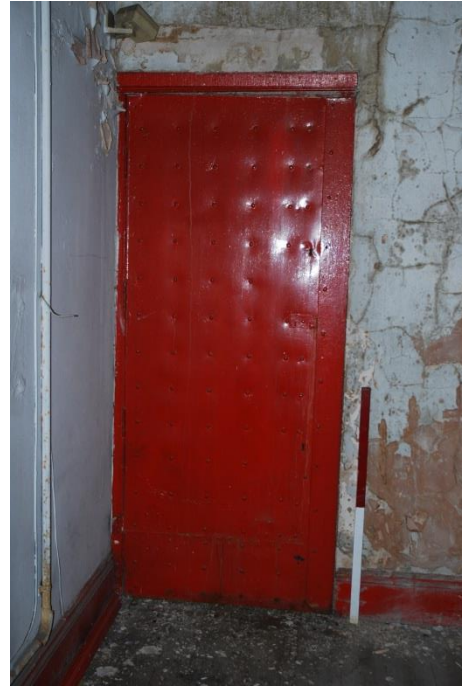
Fig 20: The strong-room door in EF61; scale 1m
