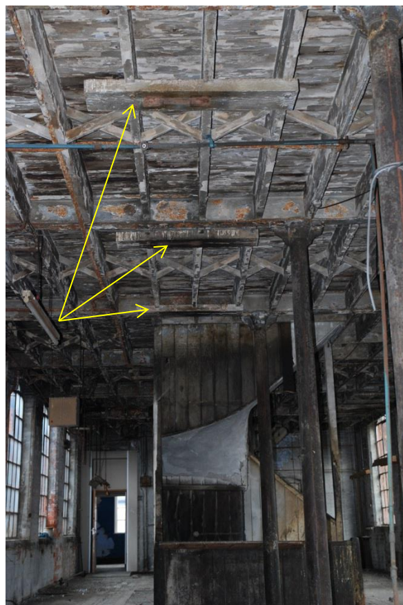
Fig 58: EF47 Drive shaft cradle remains (arrowed) showing how the inner ends of the shafts must have terminated either side of the stairs.
