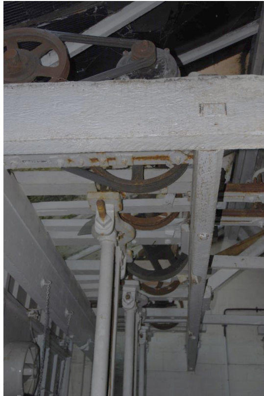
Fig 106: The timber cradle for the line-shafting of the stamp battery in EG25. The drive wheel and belt is at the top left corner (motor out of picture). Note the cast iron brackets to which are fixed the drop-press guide runners.
