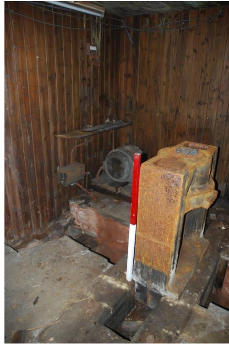
Fig 84: The press; scale 1m. Note the small electric motor behind
