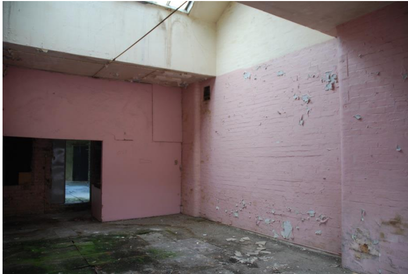
Fig 96: Rom ES21. Note the natural light from above.
