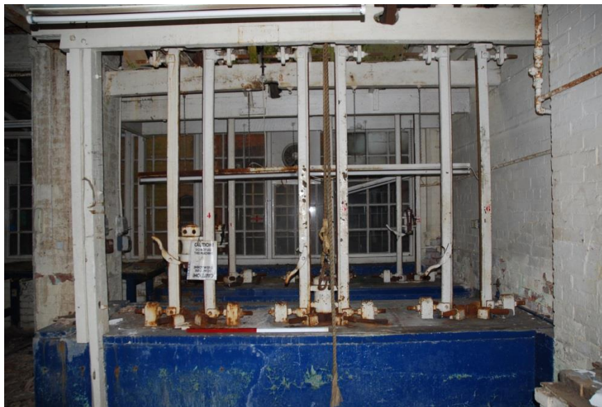
Fig 105: Surviving stamp battery in Room EG25, looking south; scale 1m. The only surviving historic features in the entire works. The blue painted areas are the brick and concrete anvil-benches.
