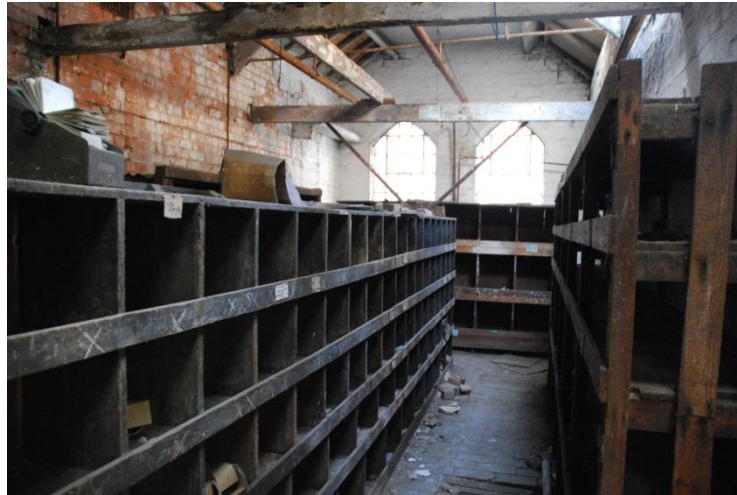
Fig 69: Room EF34 Pattern/Stock Store, looking west. The end gable walls retain line-shaft bearings.
