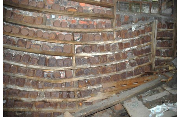
Fig 32: Stored stamps, rotting shelves buckling under their weight
