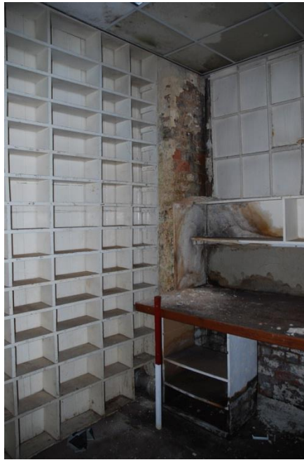
Fig 88: Room EG27 with stamp-shelves on east wall; scale 1m
