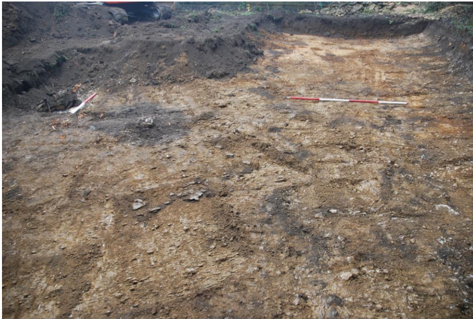
Fig 3: The site looking south, during machining; scales 2m and 1m. Note well and stump-removal disturbance at far left
