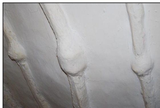
Fig 13: The rendered knots of former thatch-ties in the roof
