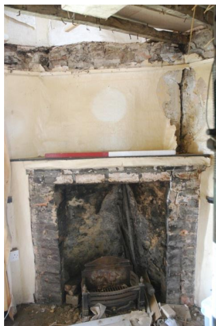
Fig 10: Inserted corner fireplace in G2; scale 1m
