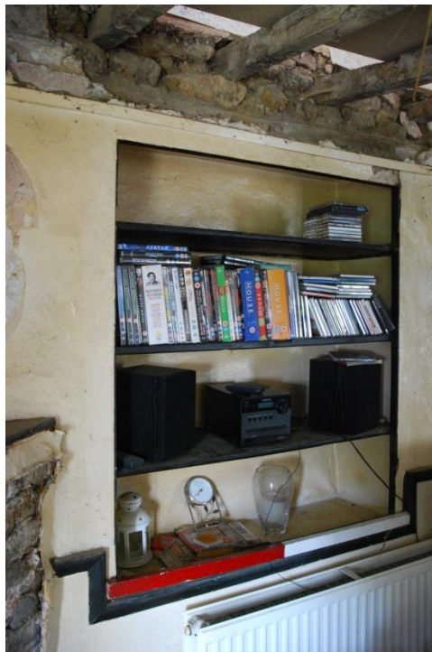
Fig 8: Blocked north-facing window in G2 – shelves on the inside; Scale 1m
