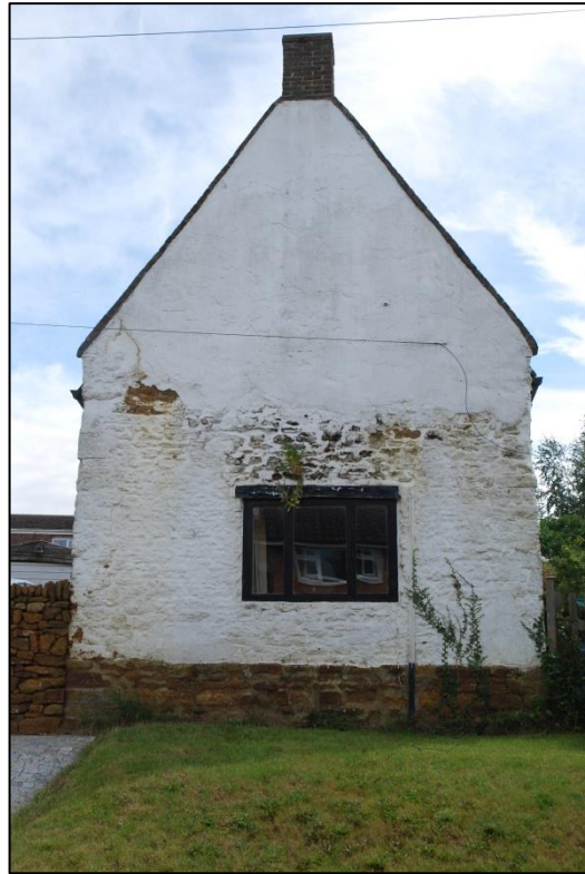
Fig 4: West-facing roadside gable-end.
