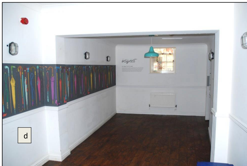
Fig 14: The extension furthest to the rear (G3), looking towards the reduced window. There may be a cellar underneath with steps down in the foreground. To left is a blocked doorway (d).
