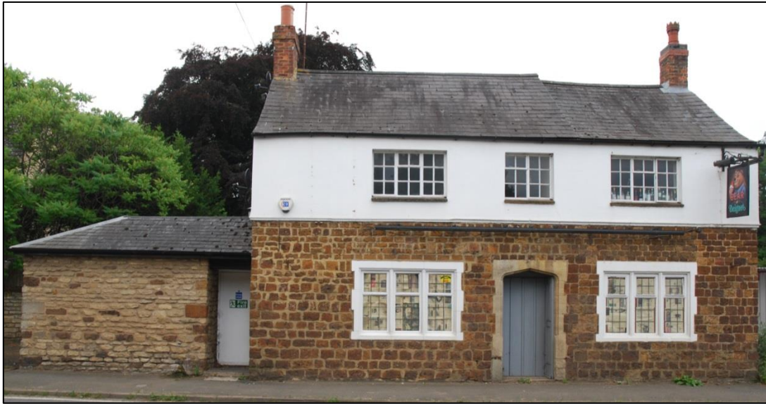
Fig 6: The roadside frontage of the pub, unbalanced by the addition of the toilets to the left. The stonework of the main frontage differs from all other faces and the fenestration reflects a 'completed' frontage.
