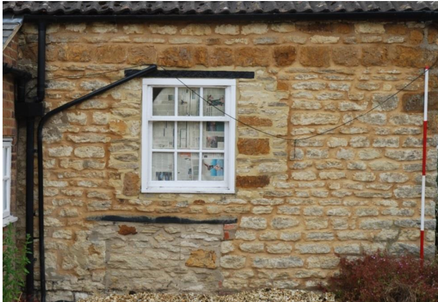
Fig 9: External evidence for a cellar – note the blocked low cellar light. Also the narrowed ground floor window; scale 2m
