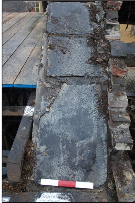
Fig 25: Slate-covered channel on interior gable for collecting and channelling smoke and steam away. Scale 30cm
