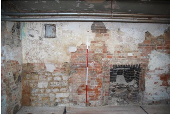
Fig 14: Middle (open) and left-hand (blocked) fireplace in B7; scale 2m
