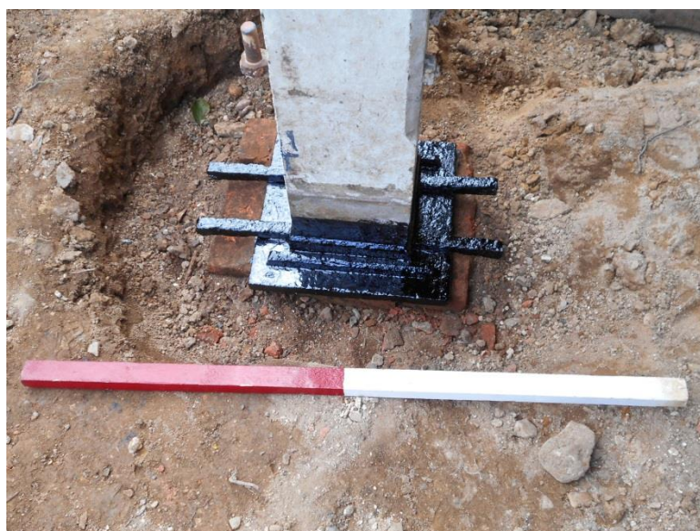
Fig 20: Cast iron pier/door-post on inserted brick base. Scale 1m
