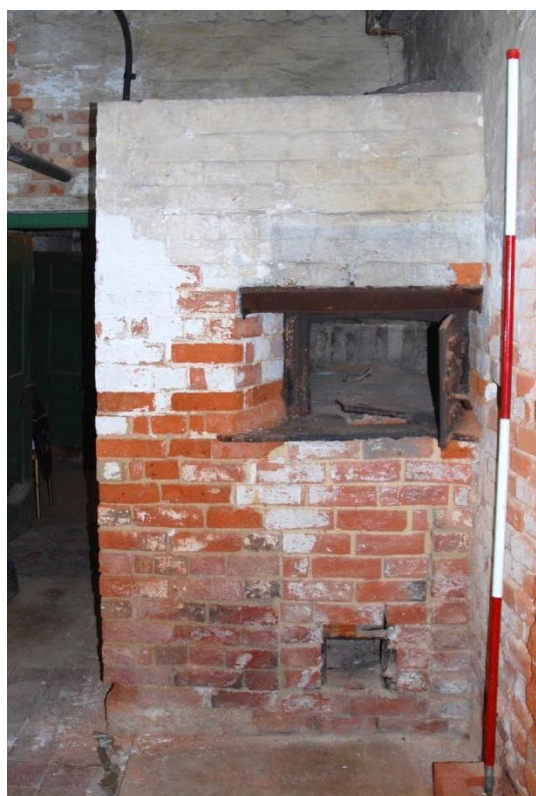
Fig 17: The secondary bread oven which dominates room B8 and which when first built, lay fully within a conjoined B7 and B8; Scale 2m. In 2016 the authors recorded the remains of an identically-sized square oven like this in Buckinghamshire dated c1842.
