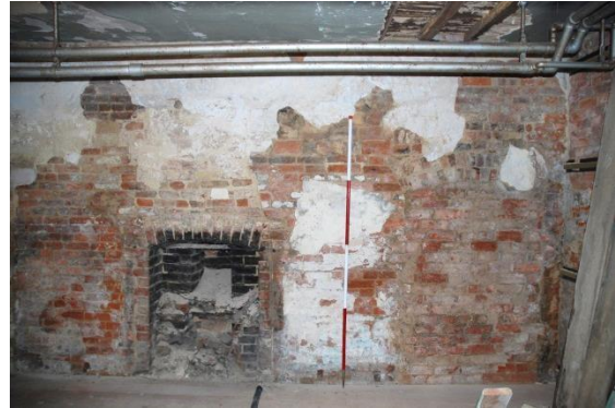
Fig 15: Middle (open) and right-hand (blocked) fireplace in B7; scale 2m
