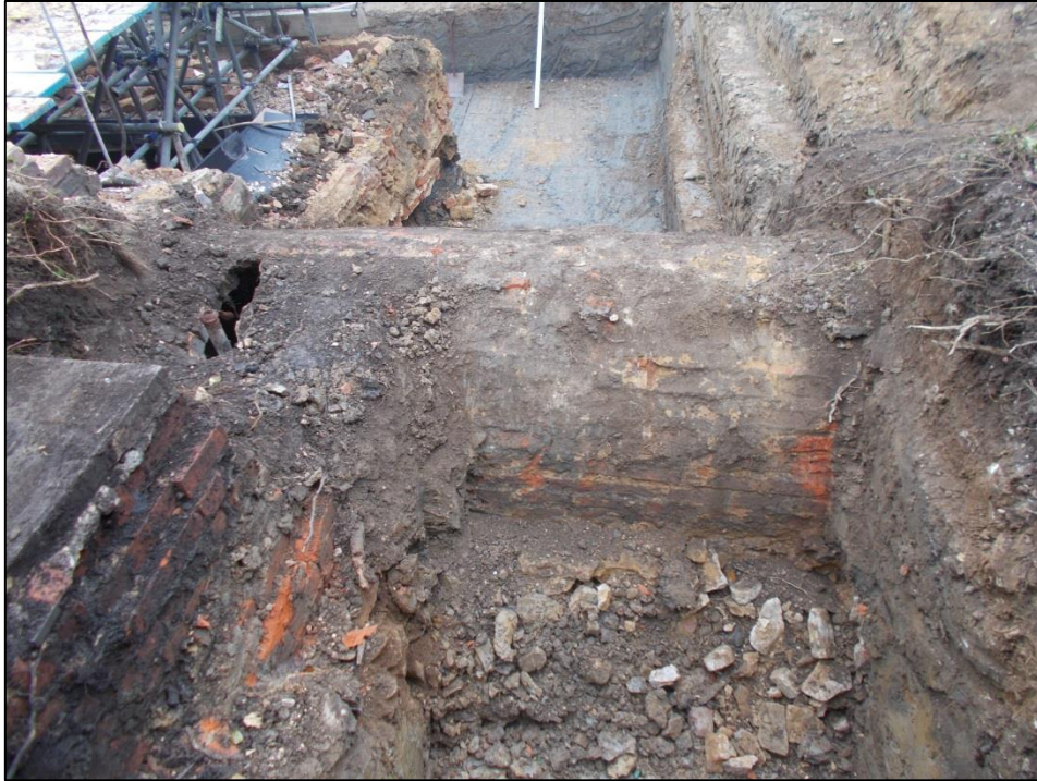
Fig 30: The tunnel vault during uncovering. Note the left-hand end breached. To left front is a later drain with inspection chamber.
