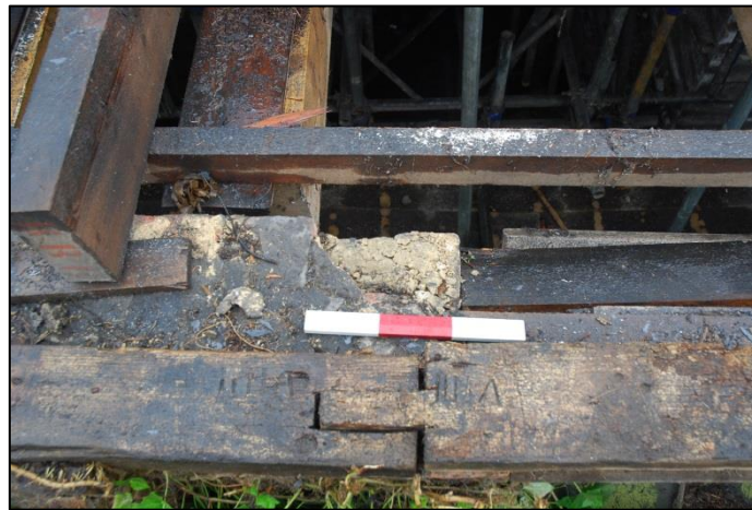
Fig 24: Scarfed sections of wall-plate with carpenter's marks (VIII); scale 30cm
