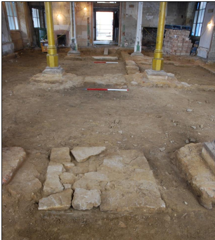
Fig 5: View looking north along the row of reduced pier-bases left over from the market hall as first built; Scales 1m
