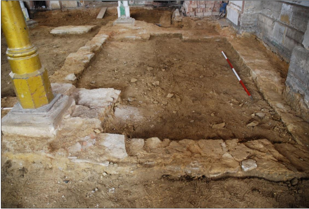
Fig 6: View looking north along the inserted 'Constable's room' of c1838; Scale 2m
