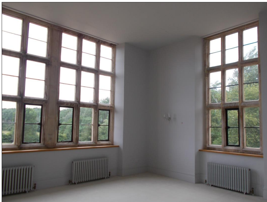
Fig 42: Room F4 with the west and north windows, looking north-west.
