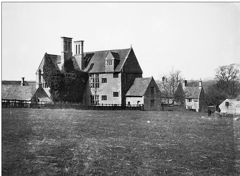
Fig 15: The house looking north-west, 1907. HEA image bb44_01106.
