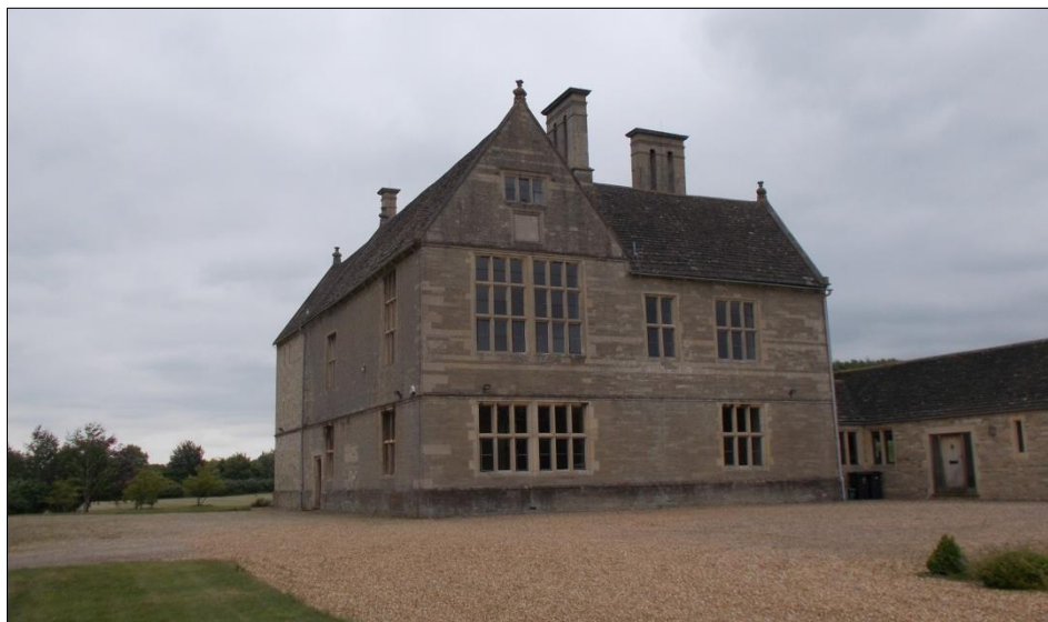
Fig 6: The same view as Fig 5 today. Former East range lost to left
