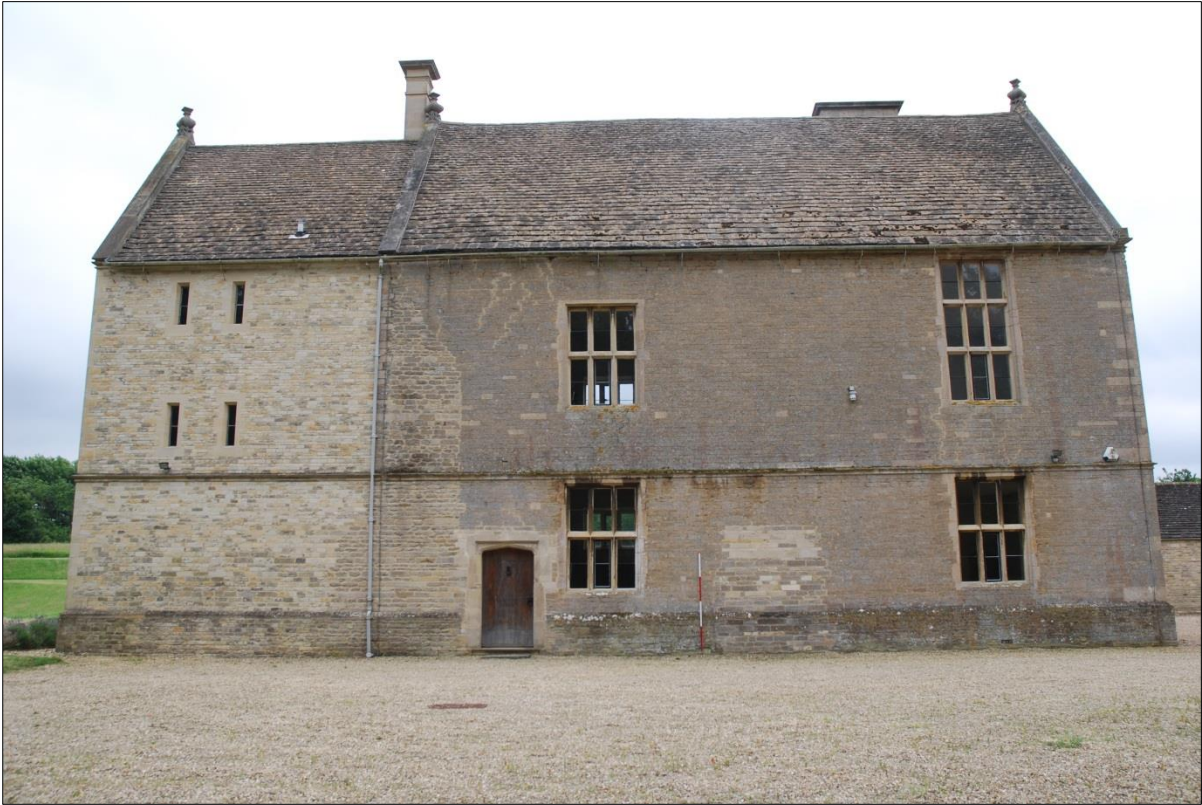
Fig 25: The north elevation. 2m scale.
