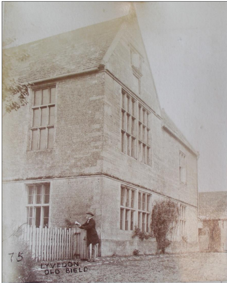
Fig 7: Photograph of 1882 showing the Old Build from the north-west (NRO: TBF277).
