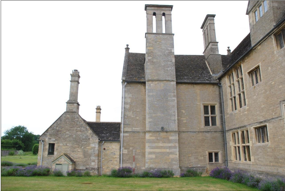
Fig 31: The east elevation of the south range. 2m scale.
