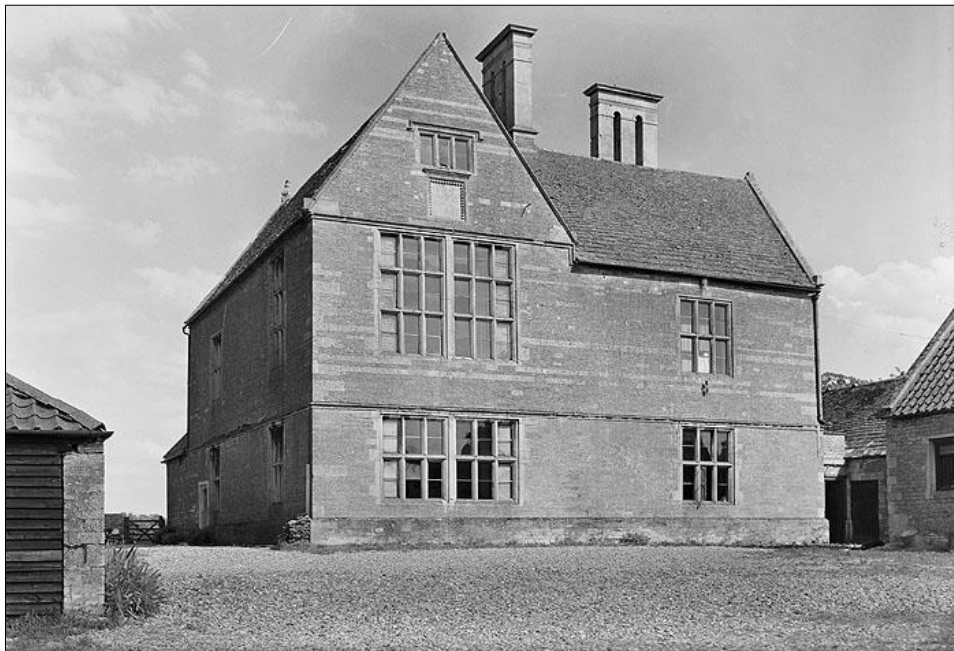
Fig 19: The house looking east-south-east in 1947. HEA image aa48_03665.
