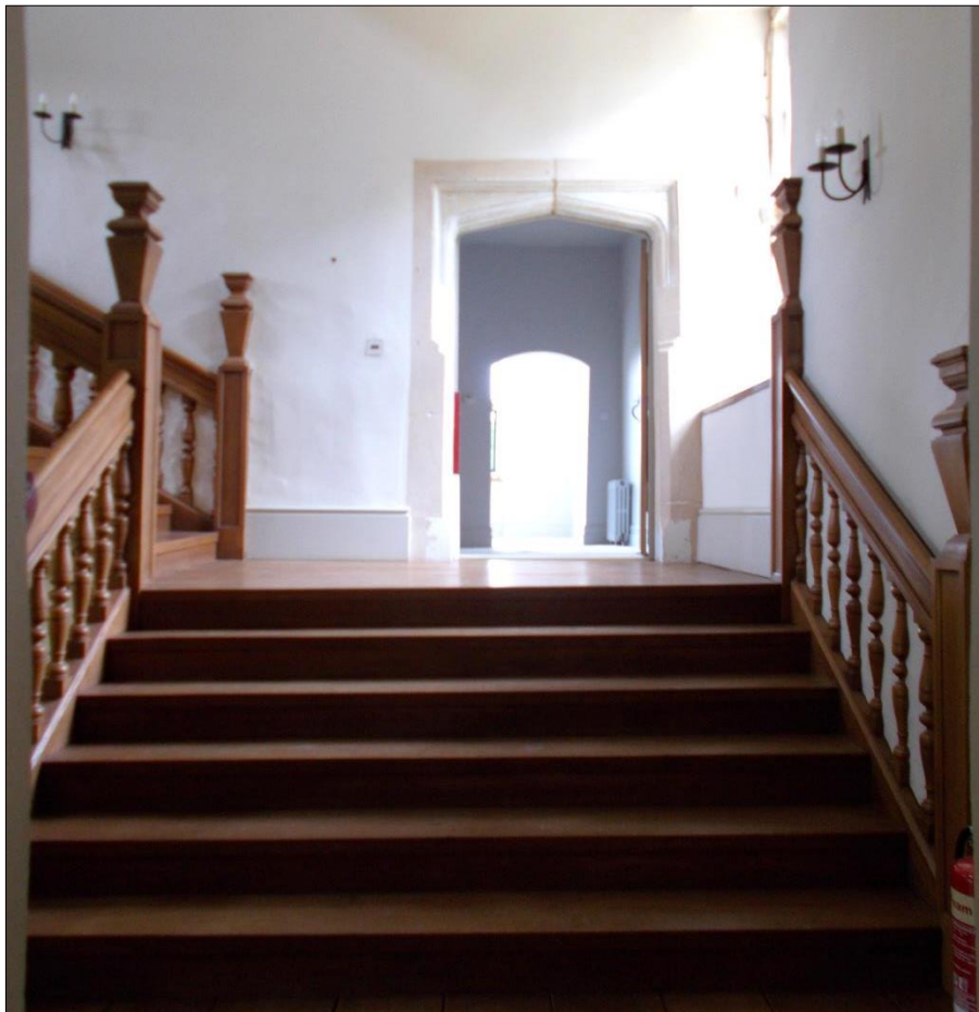
Fig 41: The wider staircase and landing leading to F1, looking west; scale 1m.
