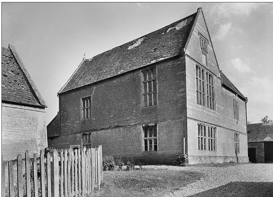
Fig 18: The house looking south-east in 1947. HEA image number aa48_03664.
