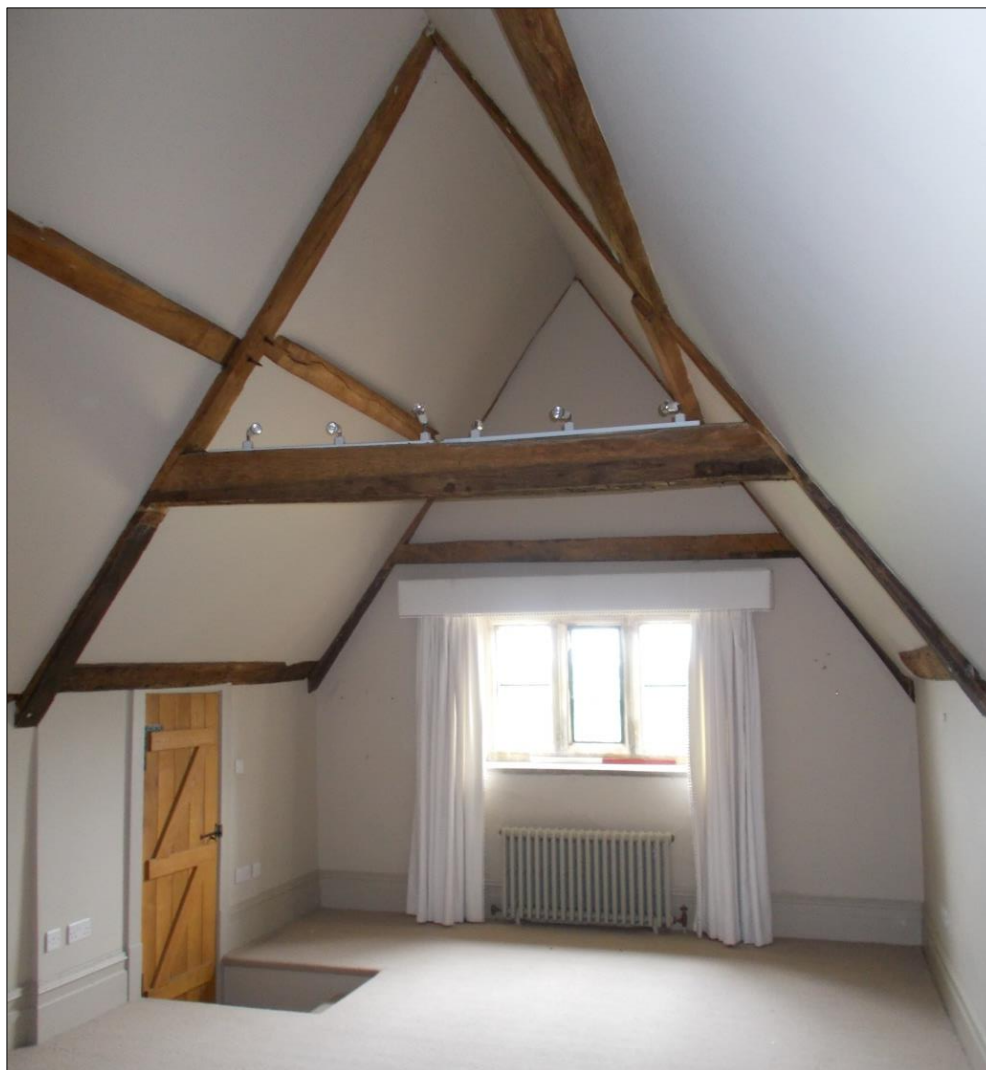
Fig 45: Room S4, looking west.
