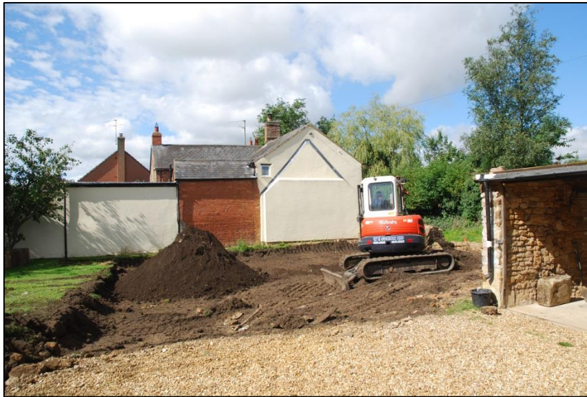
Fig 5: The site looking west during machining of the topsoil; garage building to right
