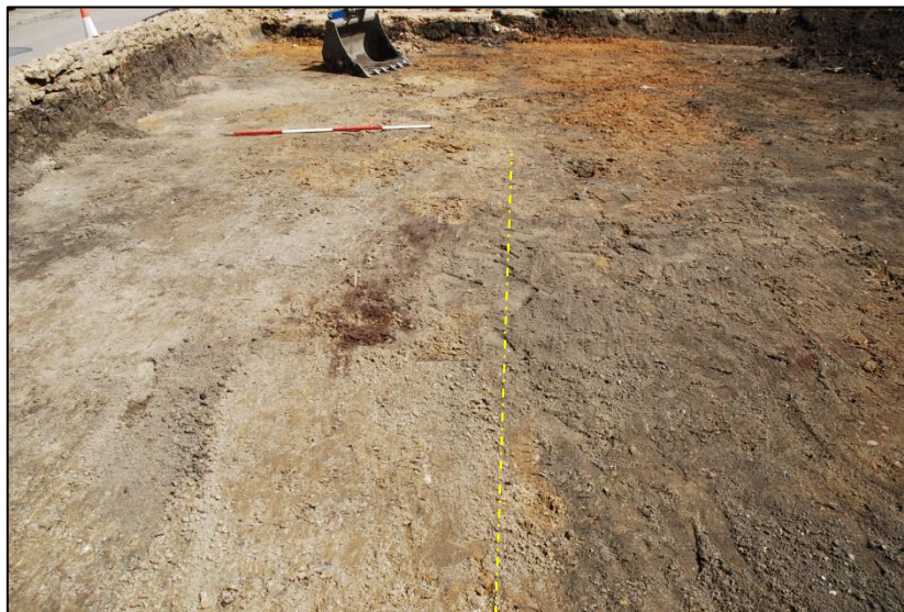
Fig 9: The site following machining, looking east. The stark difference along the dashed line is a 'mortary smudge'- all that remained of the cottage demolition (left) and clean subsoil (right). At top is exposed natural ironstone; scale 2m
