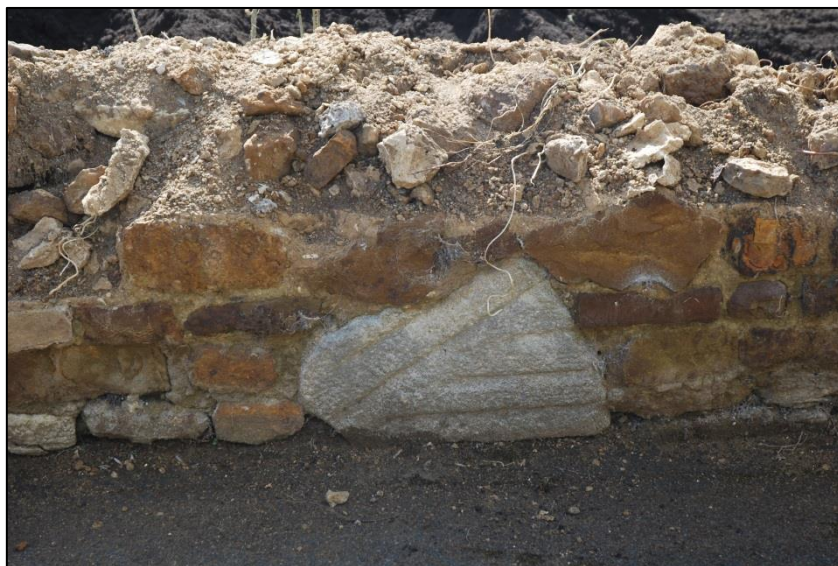
Fig 7: Broken piece of millstone re-used in the existing frontage wall
