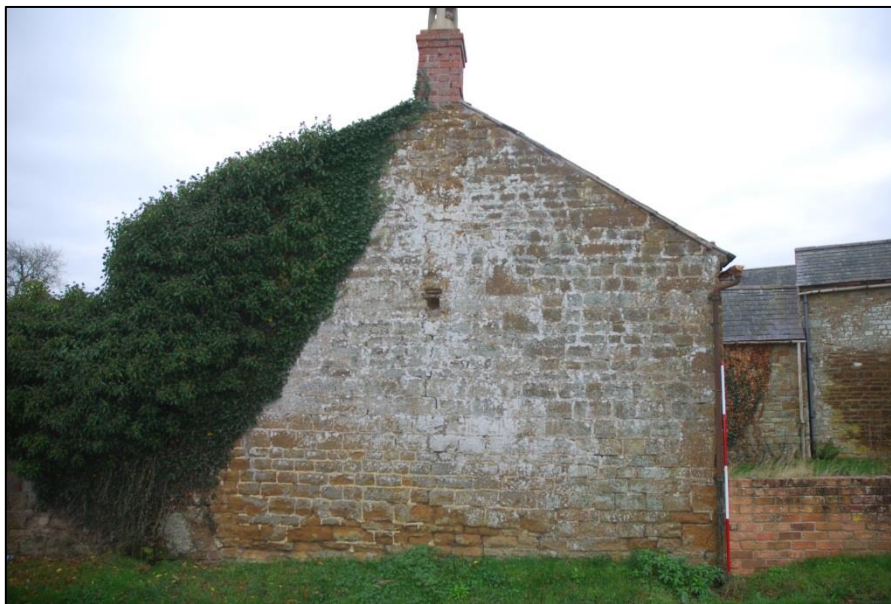
Fig 7: The north, roadside gable (scale 2m)
