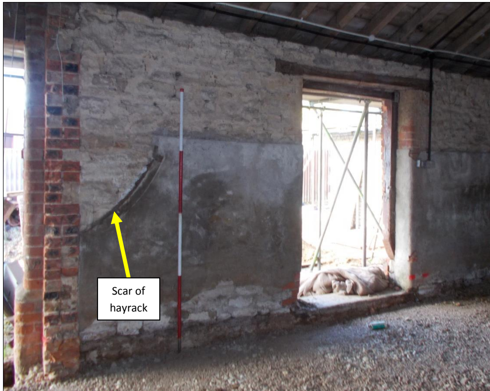
Fig 11: The former room in Barn 3 with the scar of the corner hayrack, looking north-west.
