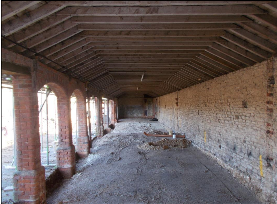
Fig 12: Barn 3, showing surviving brick piers and arches, looking north.
