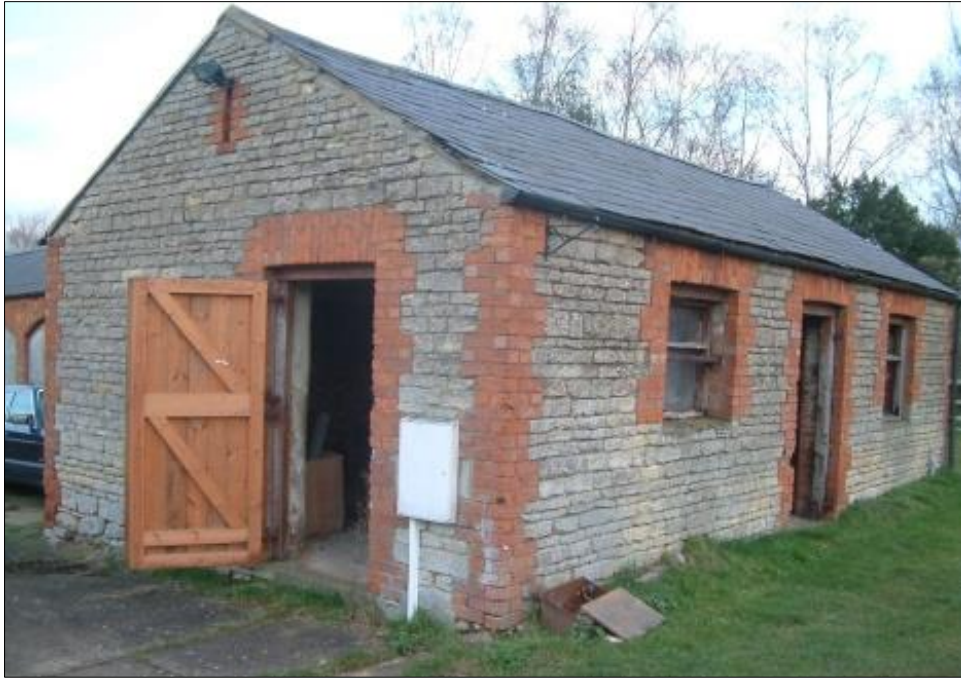
Fig 8: Barn 2, looking north-east.
