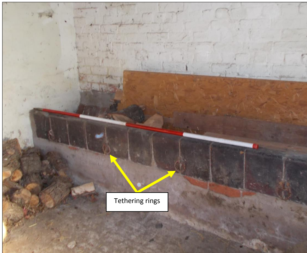
Fig 9: The manger in the west room of Barn 2, looking north-east. 2m scale.
