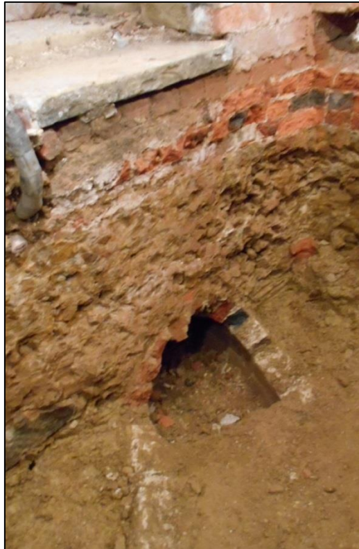
Fig 73: The library conduit where it entered from the courtyard's south-west corner, 1m below courtyard level.
