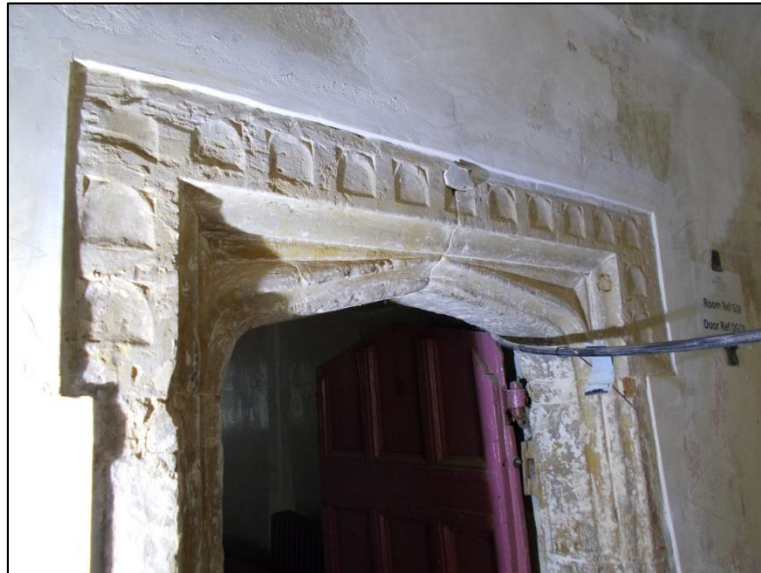
Fig 40: Fifteen tiny blind arches - stone detailing exposed for the first time for many generations in the north 'cloister'. Now believed to be possibly a monastic doorway.
