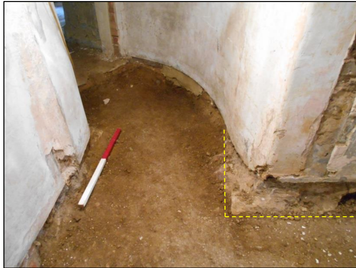
Fig 52: Floor reduction in G5; the curved corridor (looking north) shown to be an adaptation of a more angular access, linking G5 through G6 and into G7, the changes covered by render; scale 1m
