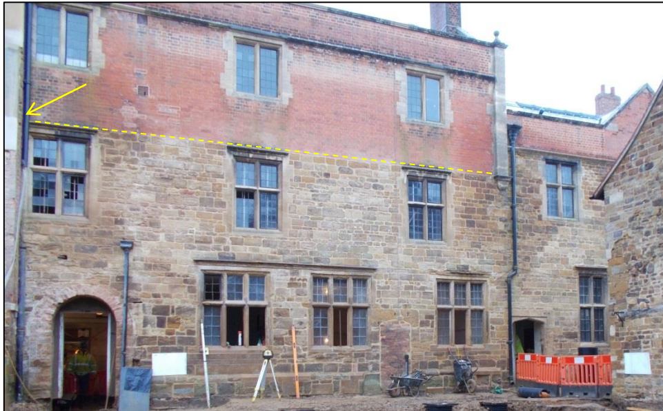
Fig 51: The majority of the East Range's east face, in a view briefly opened up by the archaeological excavations and then only possible after the scaffold cradle had been taken down. Note the added top floor in brick. The interior location of a gable kneeler (illustrated below) is arrowed. Supposed medieval doorway below.
