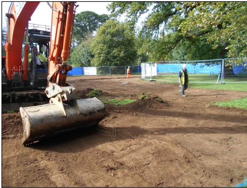
Fig 33: Stripping turf for the Car Park under archaeological scrutiny
