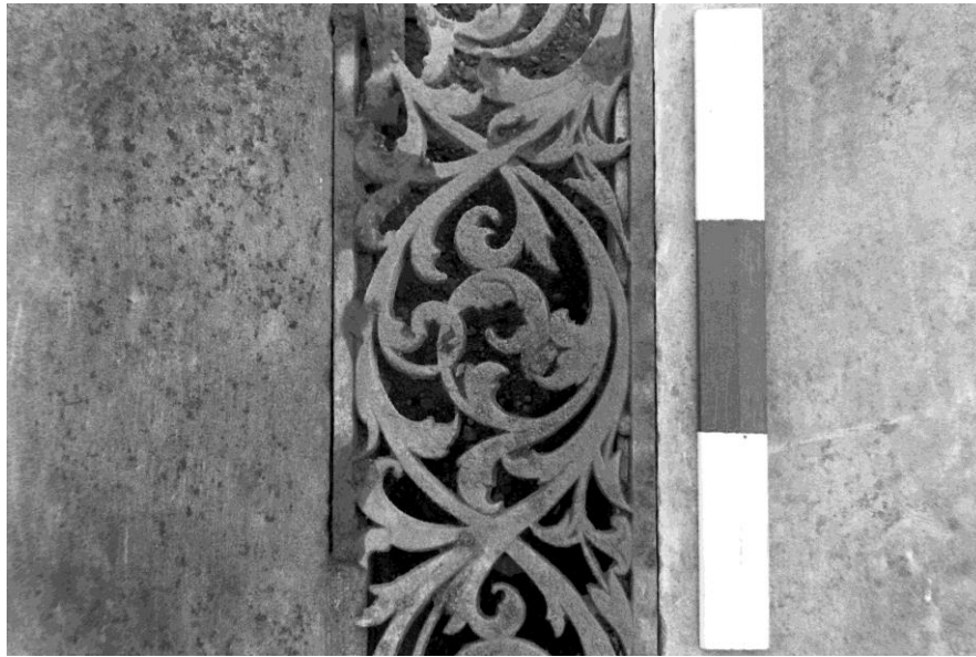
Fig 26: The elaborate cast iron grille repositioned in its rebates on broken limestone paving blocks as it would have lain in the floor over the heating pipes before demolition; scale 30cm. (Scanned from B&W negative in site archive)
