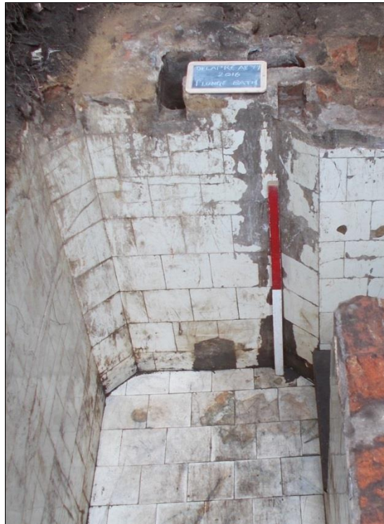
Fig 30: The former tap and drain locations in the east wall of the bath, looking east, 1m scale.
