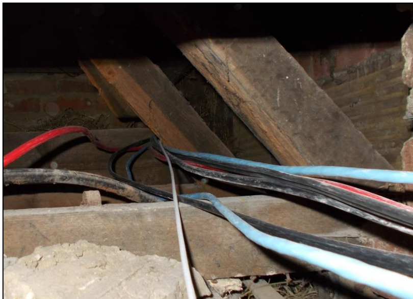
Fig 79: Glimpsed row of truncated rafters of a former, probably seventeenth-century, oak roof structure beneath the floor of rooms F23 and F24, looking west under floorboards.
