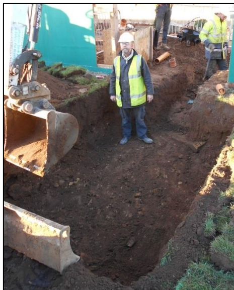
Fig 64: Digging the South Front soakaway. 1m down and still in 19 th -century material, some 5m away from the South Range. Scattered medieval architectural fragments occurred at 1.4m down.
