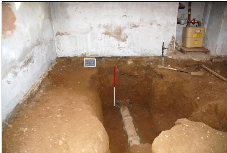
Fig 53: Floor reduction to natural geology and old services in Room G7, looking east to the outer wall. No earlier levels had survived; scale 1m
