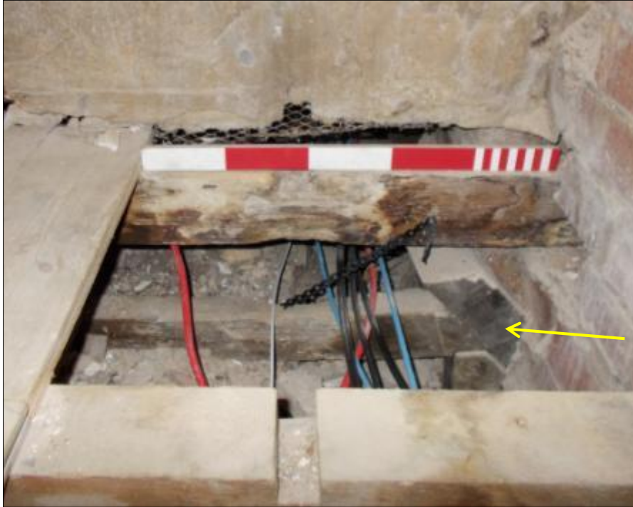
Fig 78: Sawn off rafter beneath the floor of F23 (arrowed); scale 50cm
