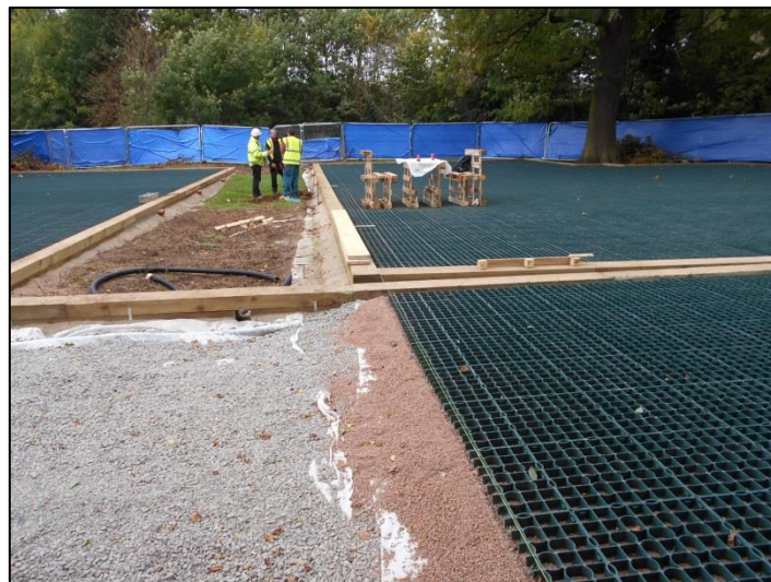
Fig 35: The car park construction mats put down over the turf-less soil
