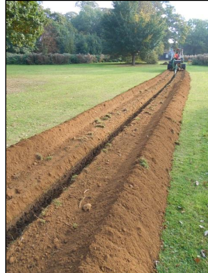
Fig 4: Use of a chain-trencher to minimise impact
