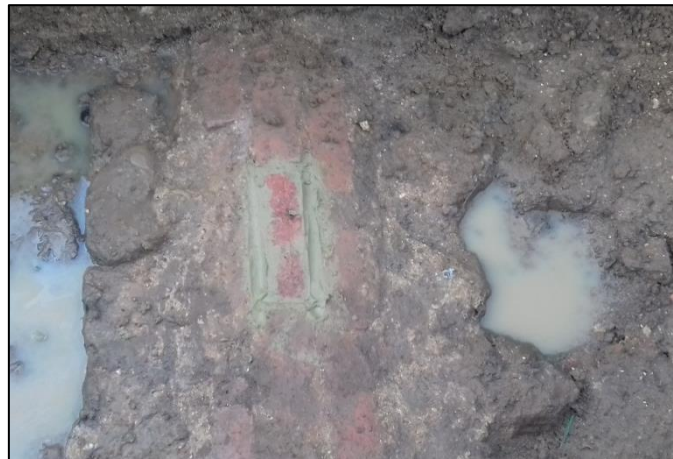
Fig 9: The inspection hole in the vault made-good
