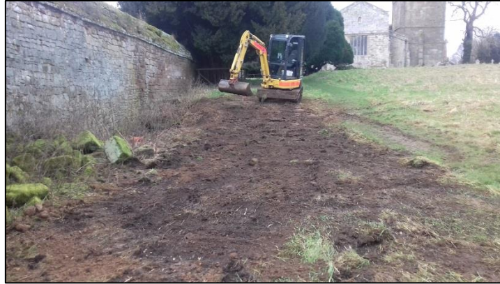
Fig 10: The trench backfilled, looking west
