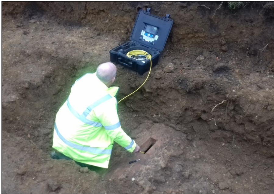
Fig 8: camera-probing the culvert interior.
