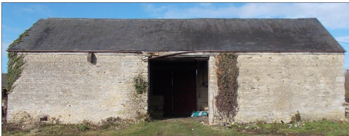
Fig 6: The east elevation, looking west. 2m scale.
