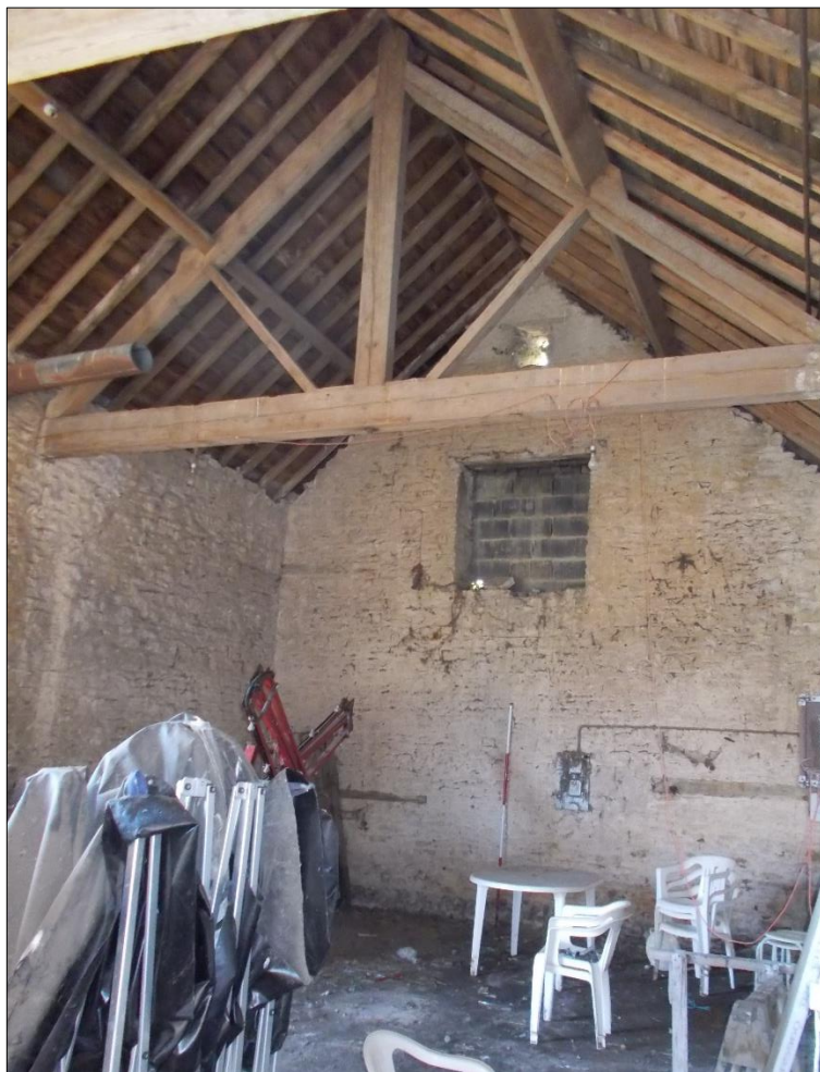
Fig 10: The south gable with hayloft door or window. 2m scale.
