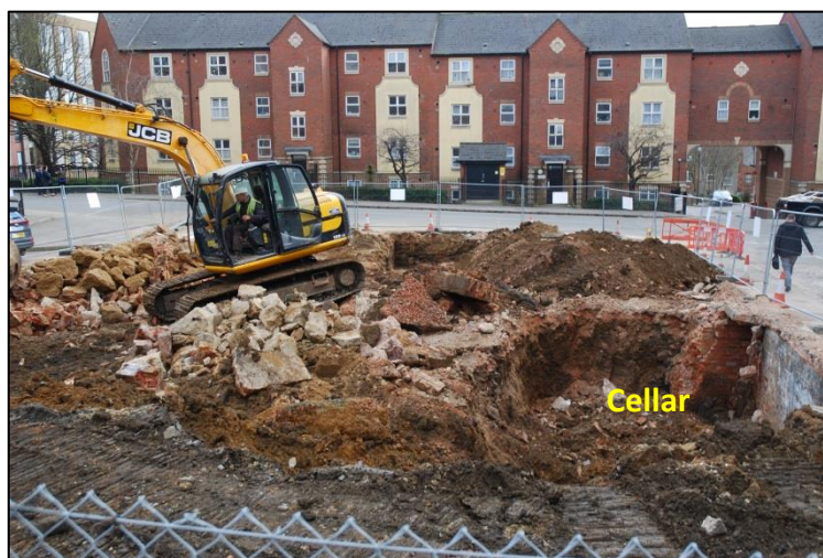
Fig 3: The site during breaking-out of floors and sub-surface impediments, looking south.
