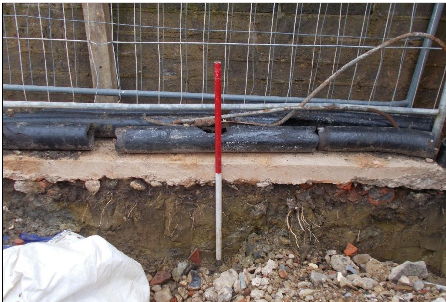
Fig 6: A remnant of the previous concrete surface and hardcore lying directly on top of the natural clay geology, looking south. 1m scale.
