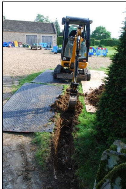
Fig 6: Machine trenching across the manor yard; garages in the background
