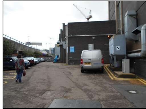
Fig 14: ...but (looking south) is riven with many buried services dog-legged out to avoid the basements
