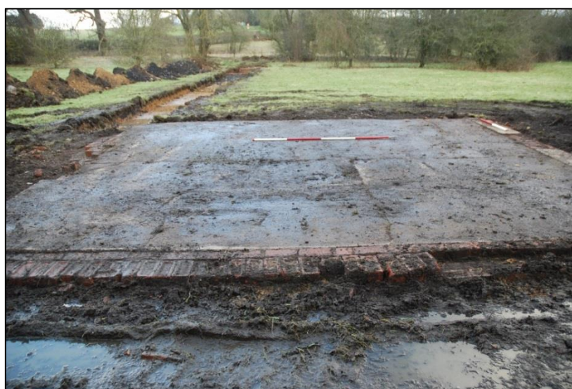
Fig 18: The concrete floor and frogged brick foundations of a small railway building which stood in the Charwelton goods-yard. It is seen in the historic photograph at fig 12 of Walker (2015). Scales 2m and 1m, the latter at a doorway in the south wall
