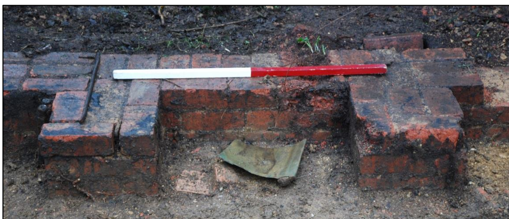
Fig 25: The brick piers and probable earth-plate; note disconnected armoured cable ends at left. Scale 1m
