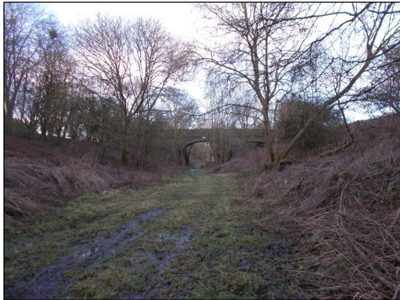
Fig 3: The abandoned cutting at the Catesby end, looking away from the tunnel mouth
