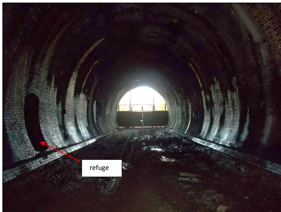
Fig 12: The northern (Catesby) end of the tunnel, looking north. Note arched refuge to the left and built-in opposed ledges which elsewhere are mostly covered in gravel.
