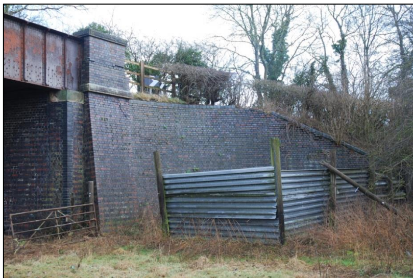
Fig 17: Staffordshire blue engineering brick bridge abutment, looking north-east
