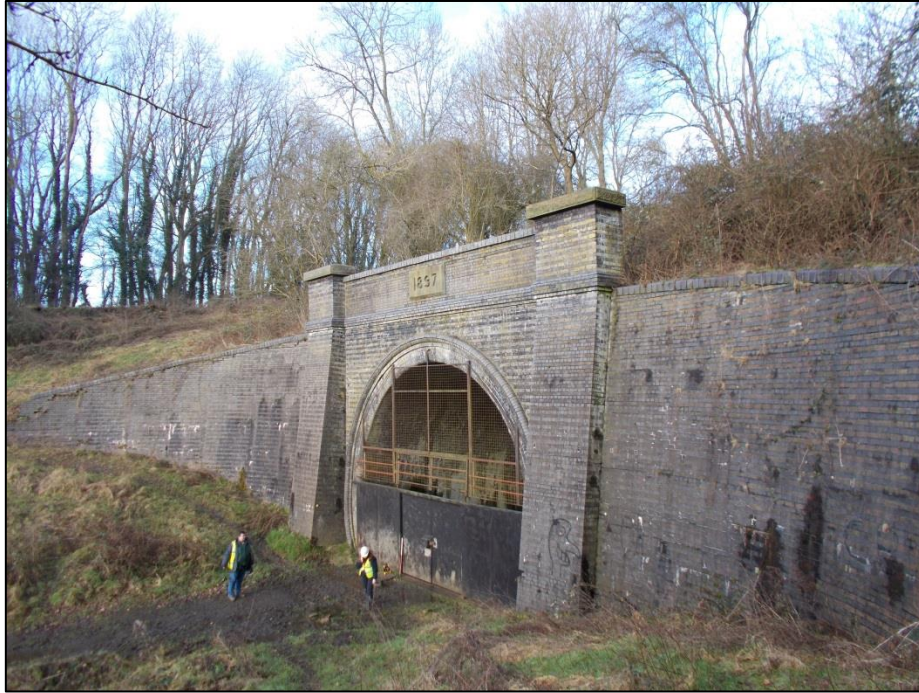
Fig 4: The southern, Charwelton-end mouth of the tunnel, with date-stone 1897.
