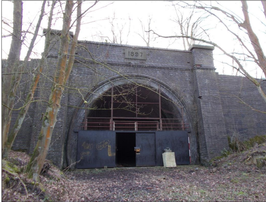
Fig 13: The northern (Catesby end) mouth of the tunnel, with date-stone 1897, looking south. 2m scale.
