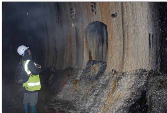
Fig 14a-c: Some of the mineralogical deposits formed in the abandoned tunnel, a by-product of water ingress
