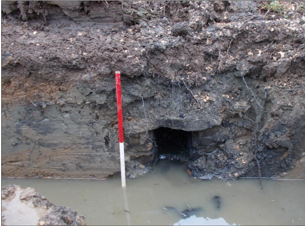
Fig 7: The stone culvert, looking north. 1m scale bar.
