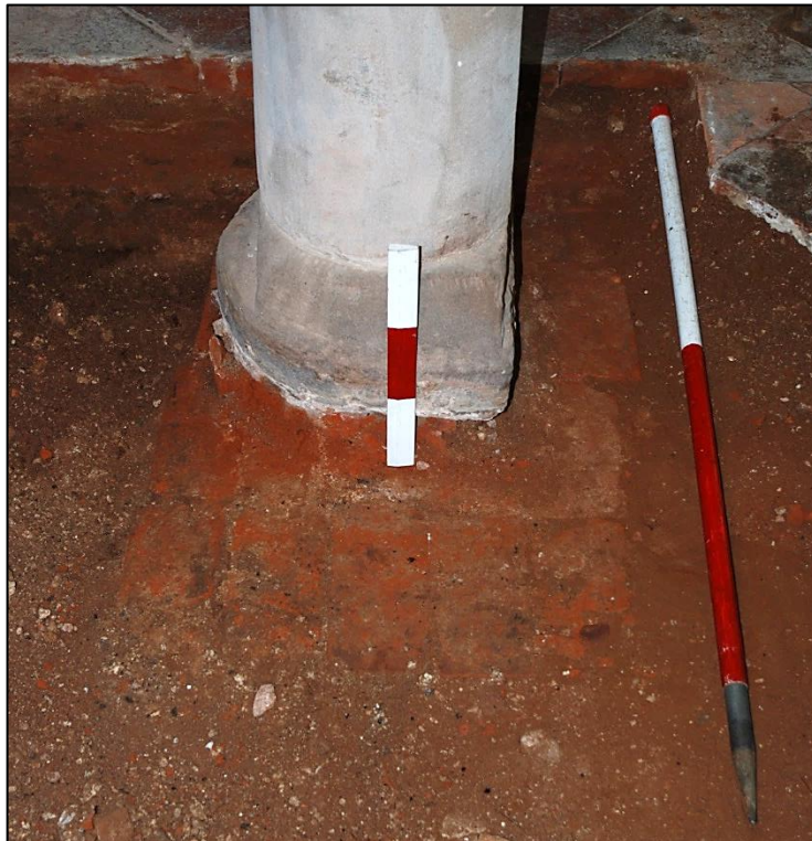
Fig 7: The brick base to the gallery pillar, showing how off-centre it is, looking north; scales 1m and 30cm
