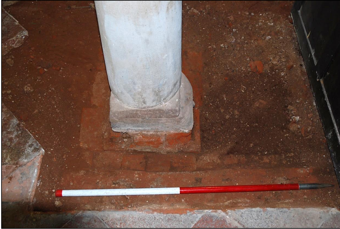
Fig 6: Brick base of the gallery pillar with the linear brick base on which the scale lies, looking south; scale 1m
