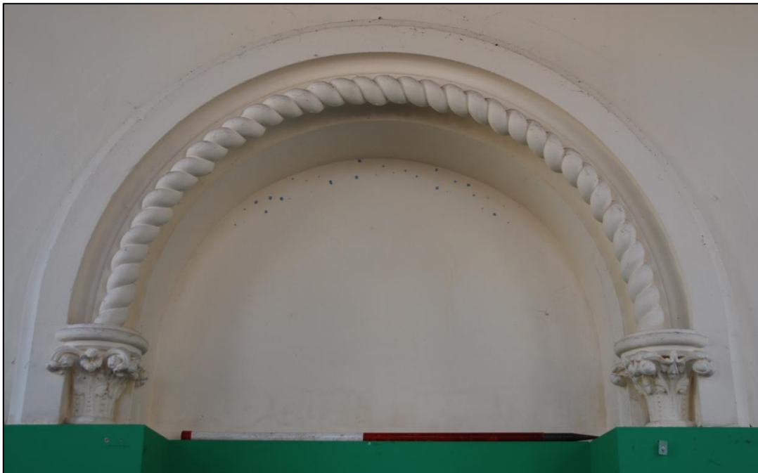
Fig 10: Round-arched alcove in the east gable framing the former pulpit location; scale 1m
