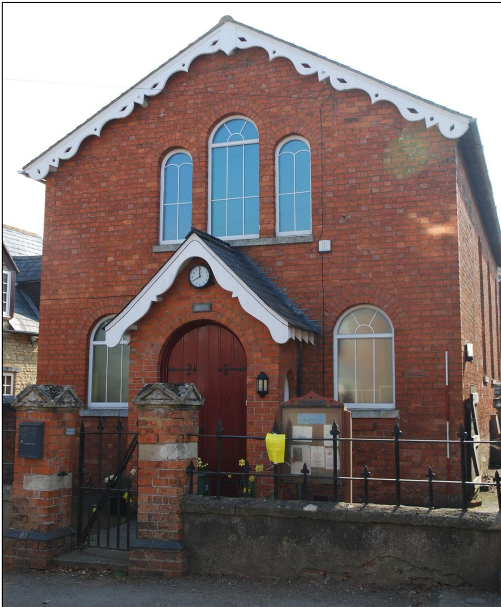
Fig 4: Street-facing west gable of the chapel, 1861 with the porch added in 1925; scale 2m
