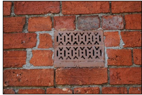
Fig 8b: Related ventilator grille, inserted.
