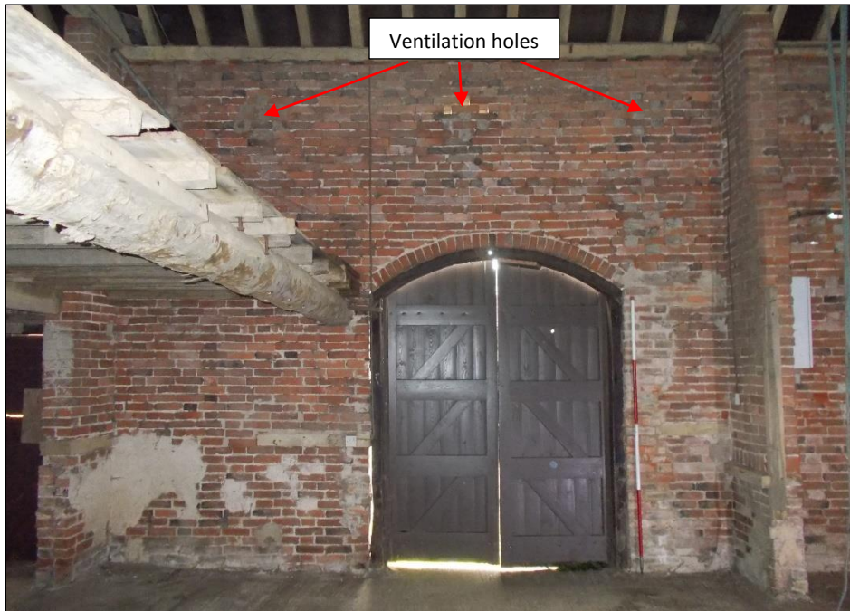
Fig 68: The central bay, looking south-west showing asymmetrical position of double-doors. 2m scale rod.
