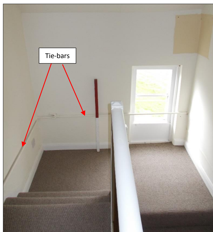
Fig 27: The upper section of the staircase, looking north-west. 1m scale rod.
