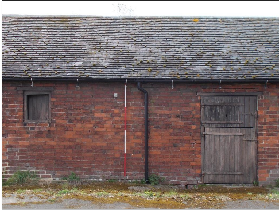
Fig 52: Room G16, former loose boxes, looking south-west. 2m scale rod.
