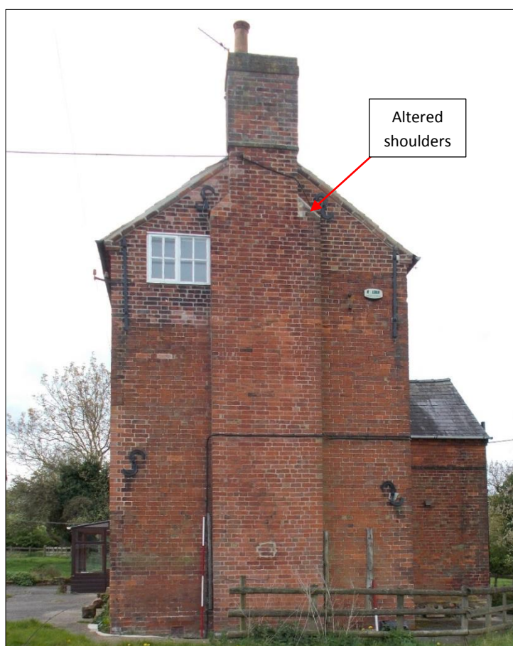
Fig 7: The north-east gable elevation, looking south-west. 1m and 2m scale rods.
