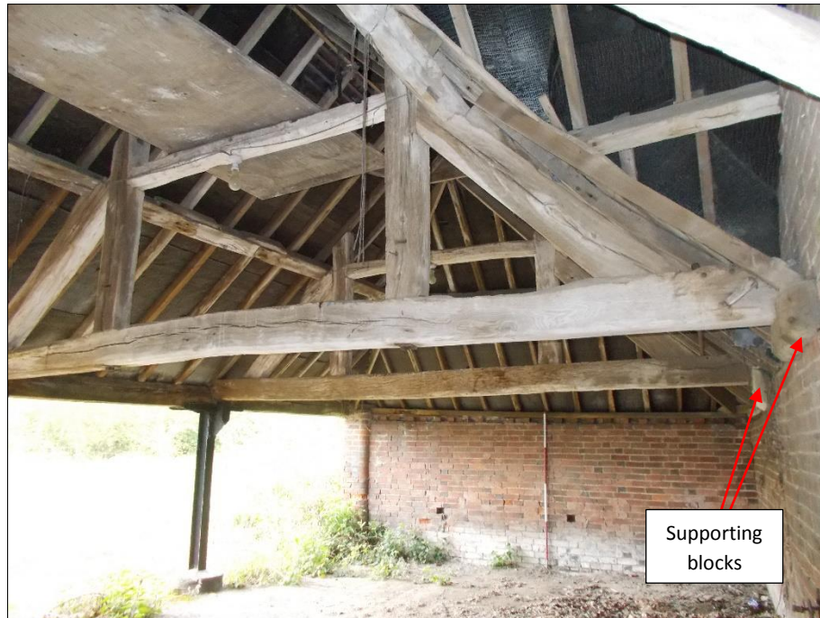
Fig 57: Room G18, the roof trusses, looking south. 2m scale rod.
