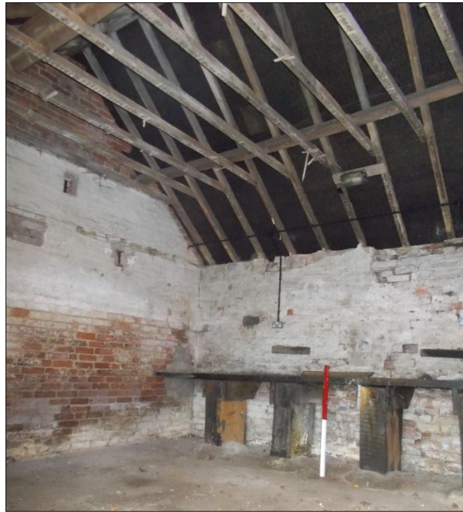
Fig 48: Room G13, looking south. 1m scale rod.
