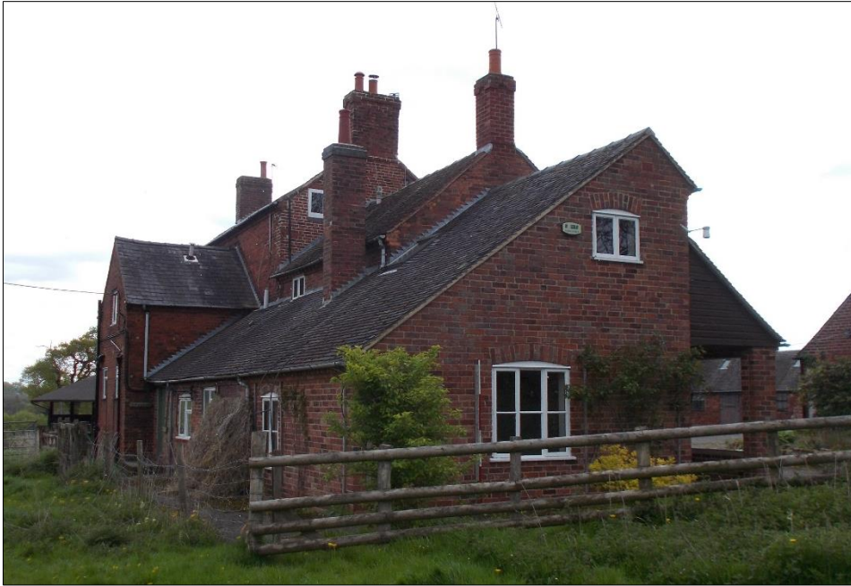
Fig 38: The late twentieth-century extension, looking north-east. 2m scale rod.
