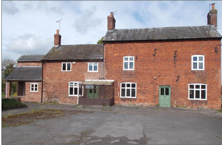
Fig 5: The principal (south-east) elevation of the farmhouse, looking north-west. 1m and 2m scale rods.
