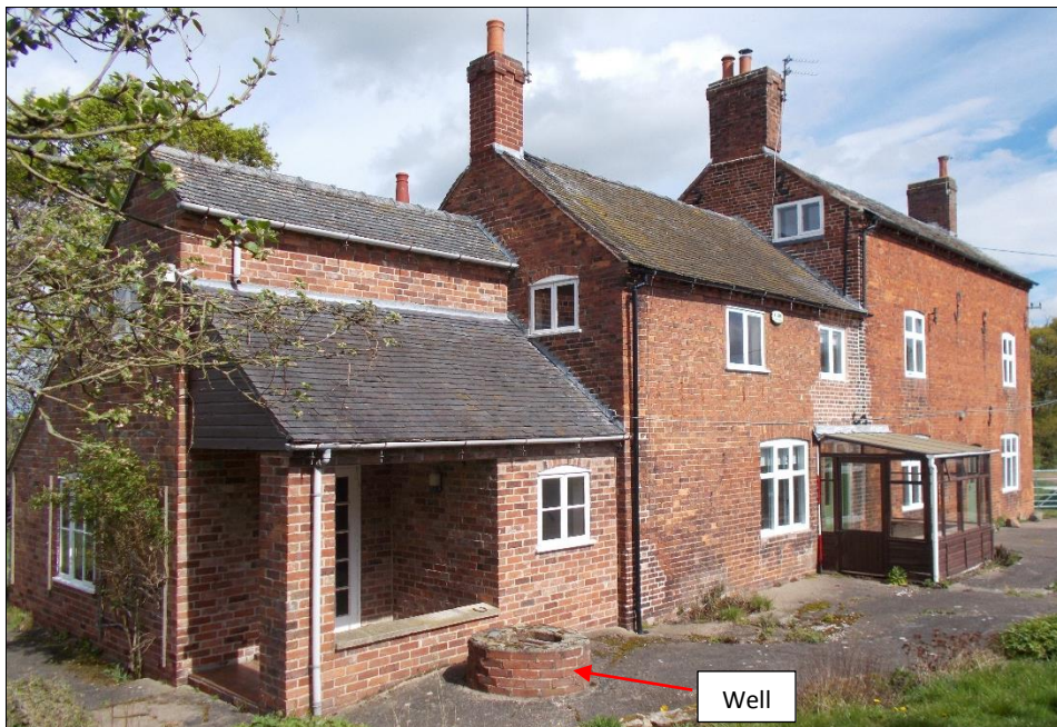
Fig 39: The late twentieth-century extension looking north. 2m scale rod.
