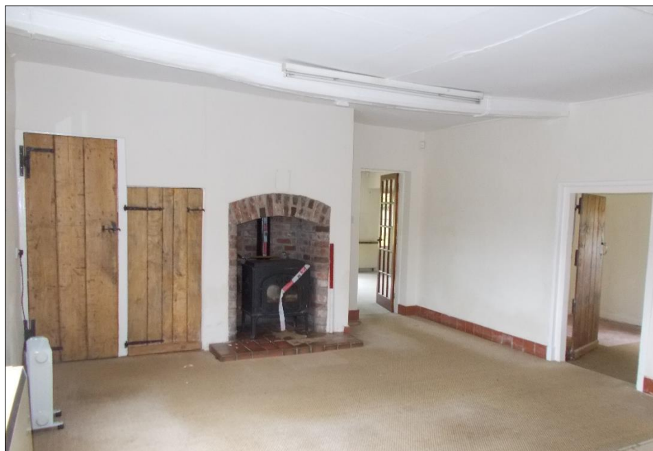
Fig 32: Room G6, the fireplace and cupboards, looking southwest. 1m scale rod.
