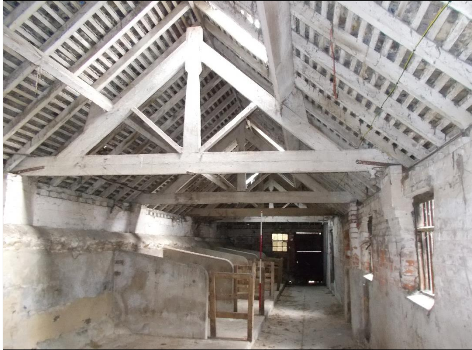
Fig 86: The cattle stall range interior, looking north-east. 2m scale rod.
