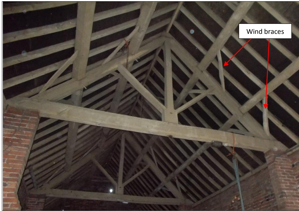
Fig 78: The barn roof, looking south-east.
