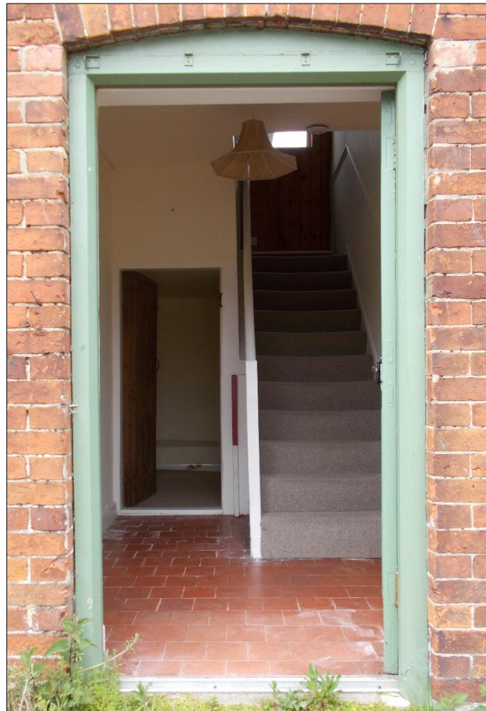
Fig 15: Room G1, the entrance hall and stairs, looking north-west through front door. 1m scale rod.
