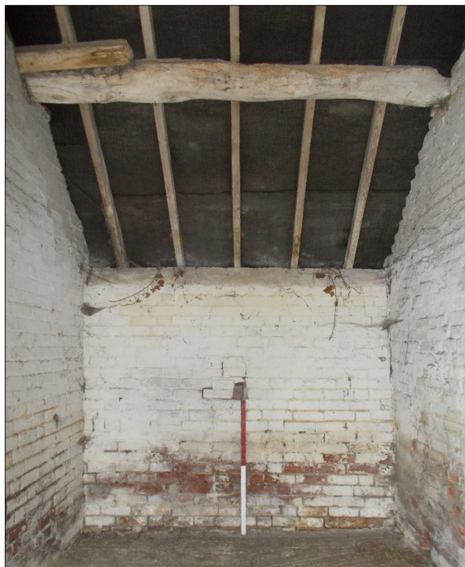
Fig 55: Room G17, looking south-west. 1m scale rod.
