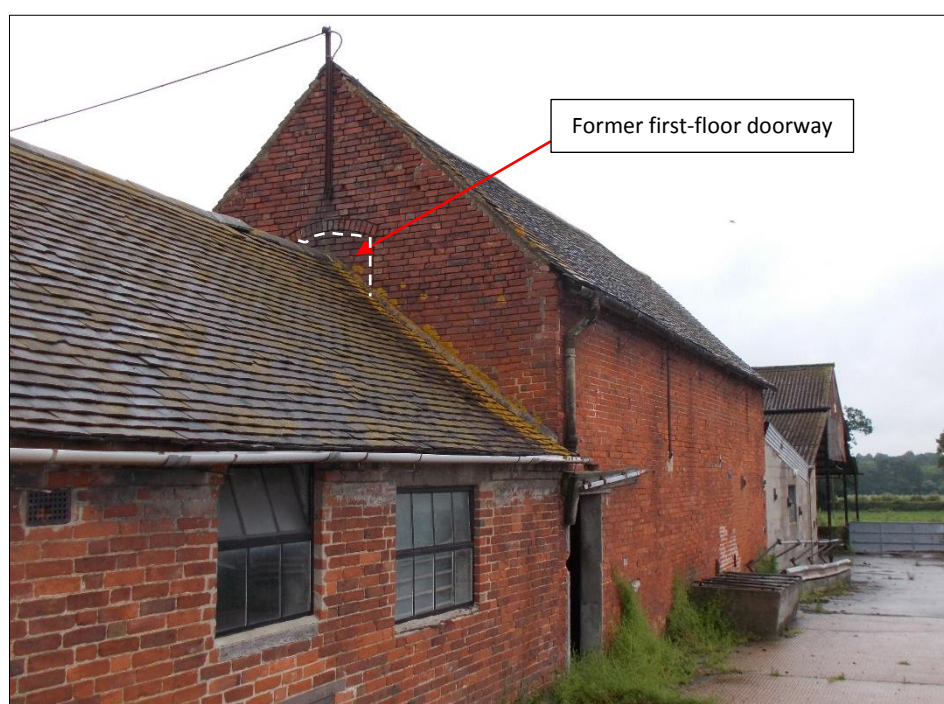
Fig 91: The southern gable wall of the two-storey dairy range, looking north.
