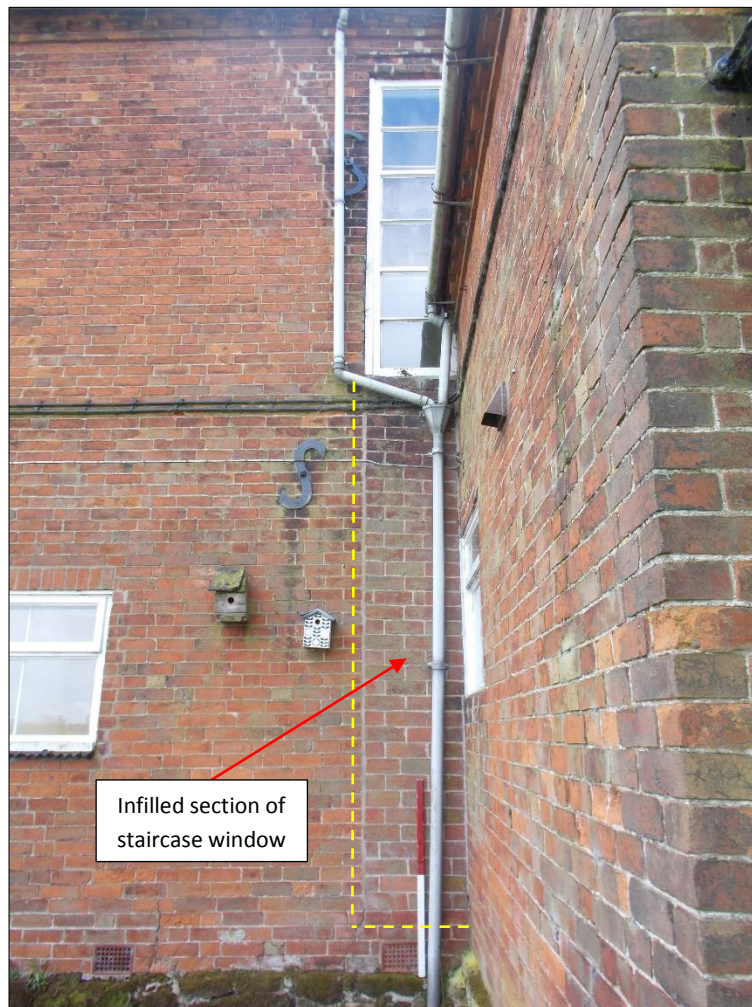
Fig 9: The partially infilled vertical stair-light, looking south-east. 1m scale rod. Note stone plinth.
