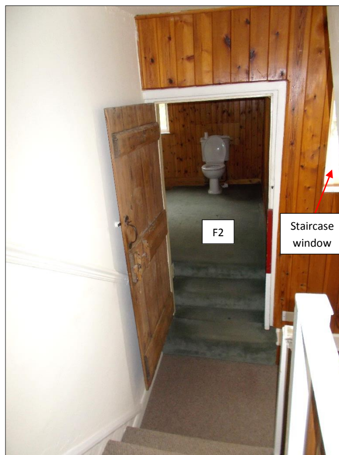
Fig 22: The half-landing, looking north-west into room F2. 1m scale rod.
