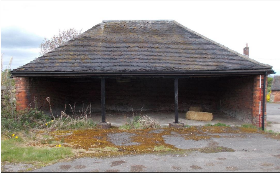
Fig 56: Room G18, the hovel, looking north-west. 2m scale rod.
