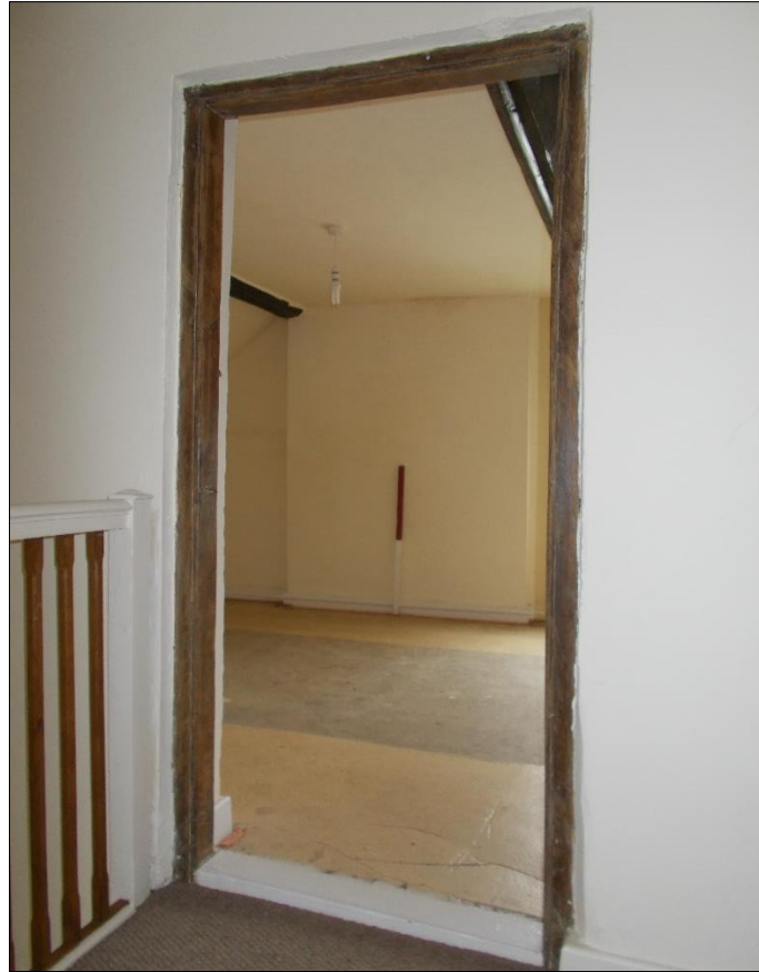
Fig 28: Room S2 looking north from the landing. 1m scale rod.
