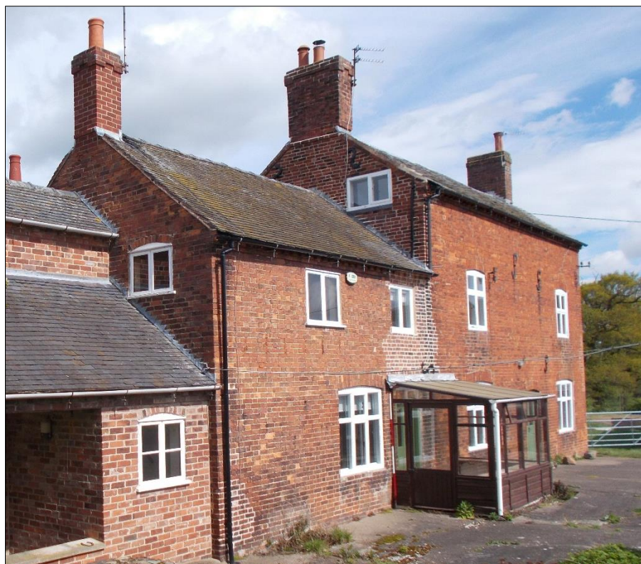
Fig 14: The phase one south-west gable looking north-east. 2m scale rod.
