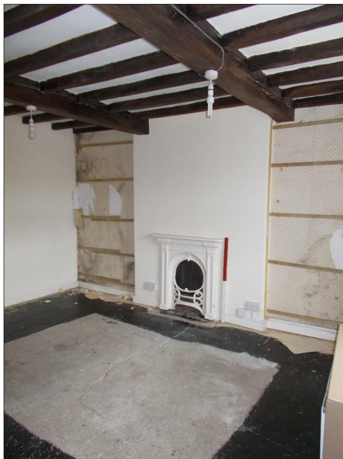
Fig 25: Room F4 looking north showing fireplace, ceiling construction and lime-ash floor. 1m scale rod.
