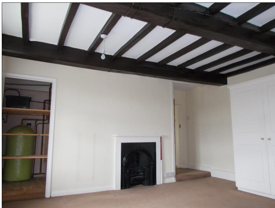
Fig 24: Room F3, the fireplace looking west. 1m scale rod.
