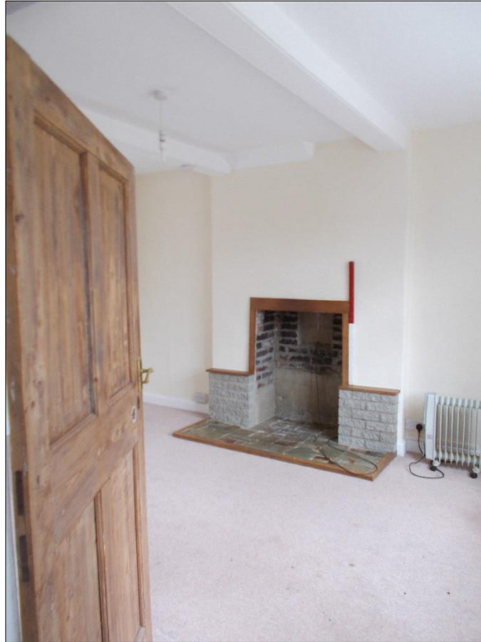
Fig 16: Room G3, the sitting room or parlour, looking north. 1m scale rod.
