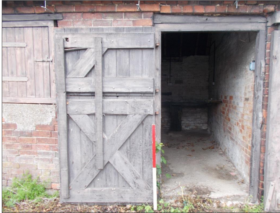
Fig 47: Room G13, the stable door looking south-west. 1m scale rod.
