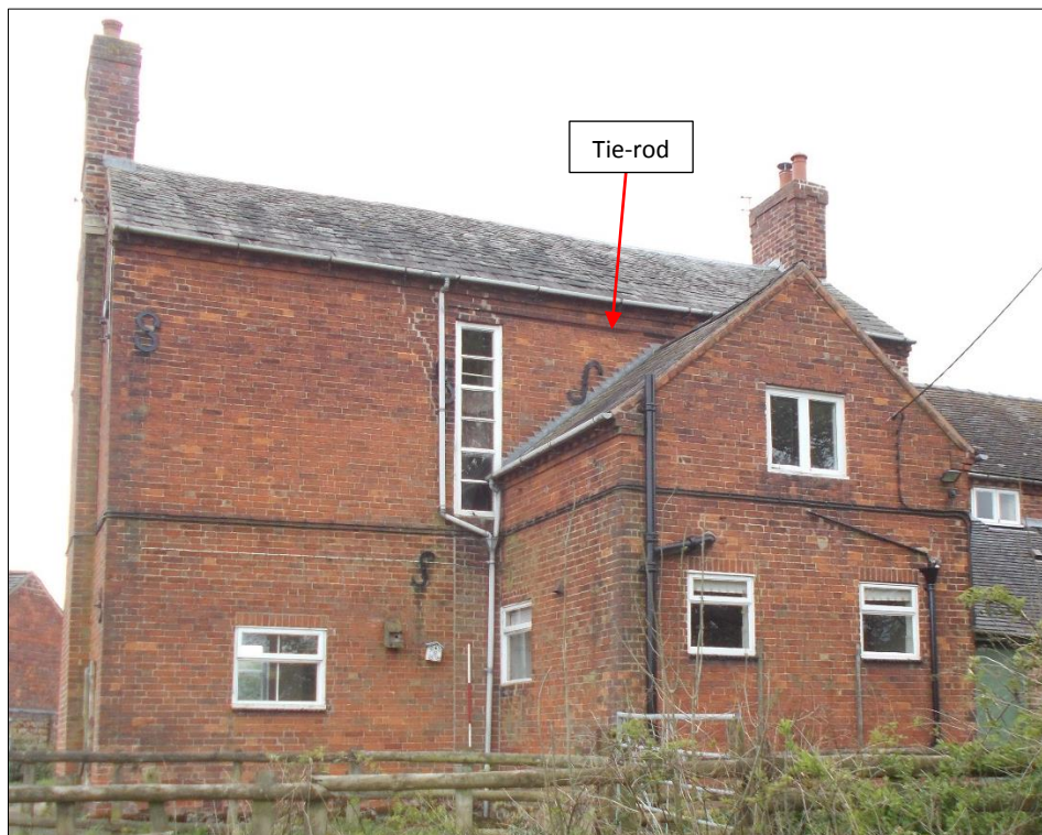
Fig 8: The rear (north-west) elevation of the 2 ½ and 2 storey sections of the farmhouse, looking south. 2m scale rod.
