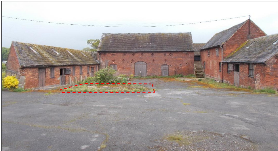
Fig 60: The stockyard barn ranges. From left to right; the cattle stalls, threshing or store barn and dairy range, looking north-east. Approximate location of lost pig-pens outlined in red dashed lines.
