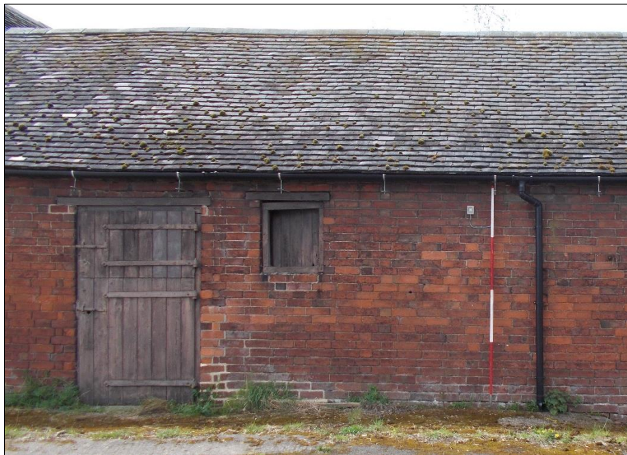
Fig 54: Room G17, looking south-west. 2m scale rod.
