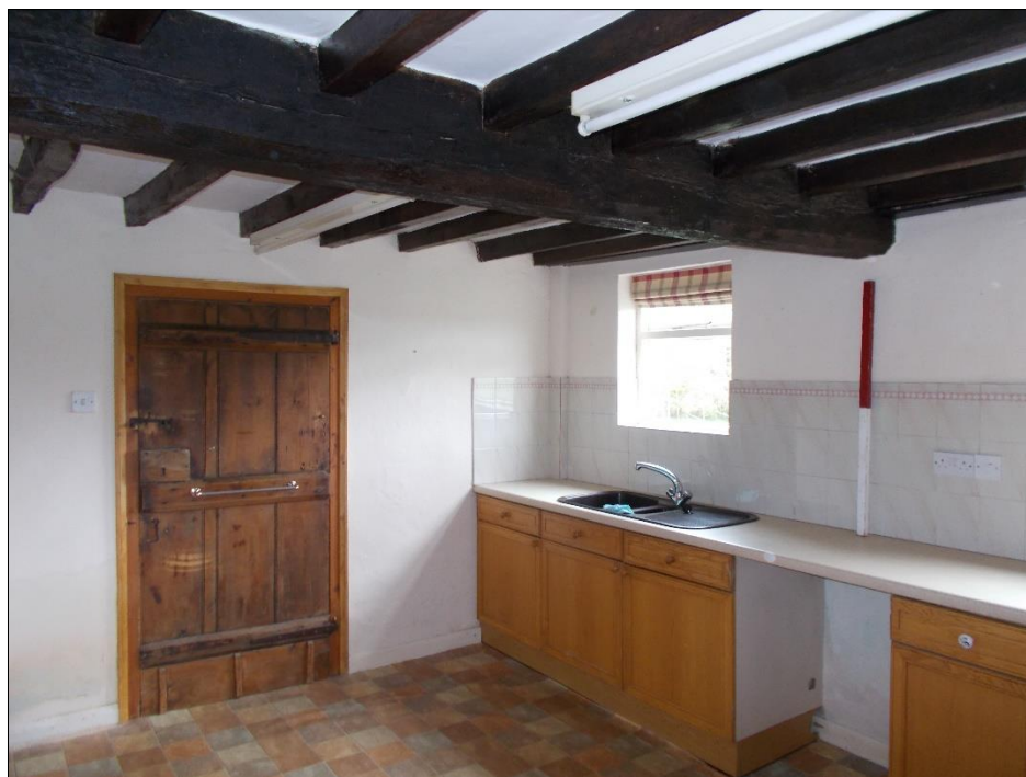
Fig 20: Room G5, the back kitchen, looking west. 1m scale rod.
