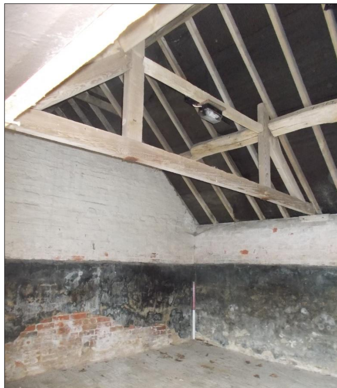
Fig 53: Room G16, interior, looking south. 1m scale rod.
