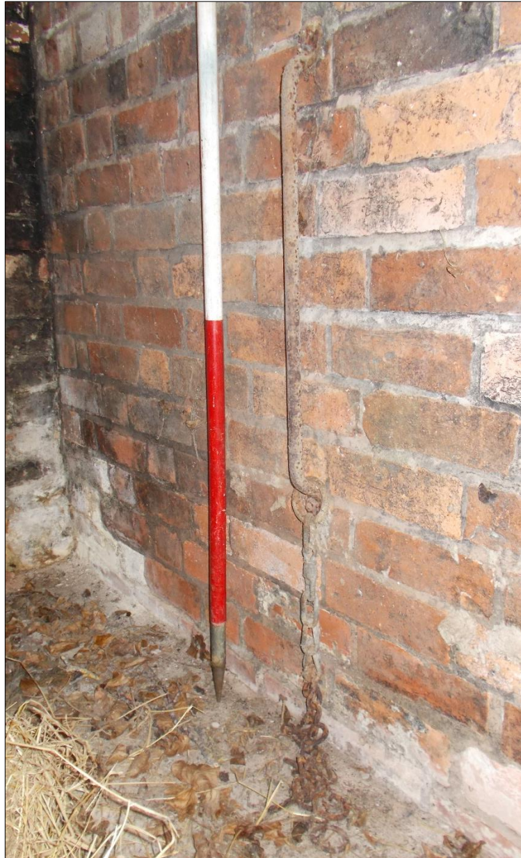
Fig 17: A tethering bar and chain in the west room of the west range. Scale in 50cm sections.
