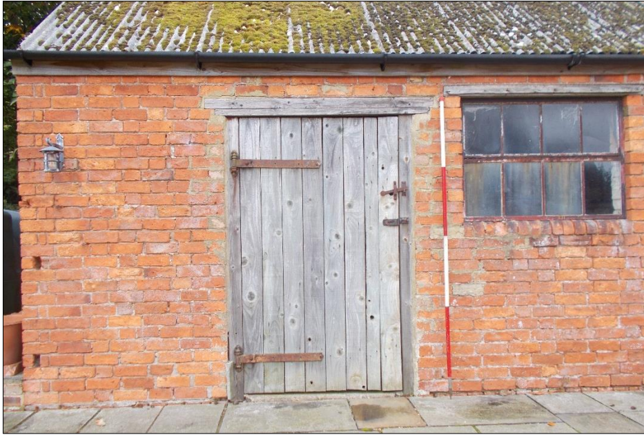
Fig 15: An example of the door and window furniture of the east range, looking north. 2m scale rod.
