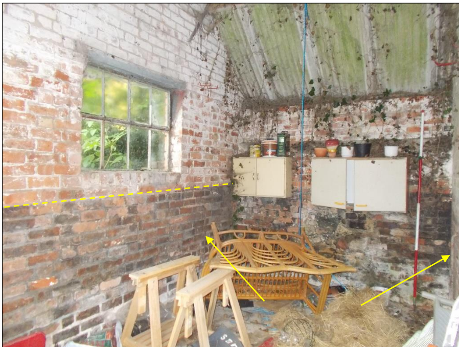
Fig 16: The west room of the west range, looking north-west. 2m scale rod. Tethering bars arrowed.
