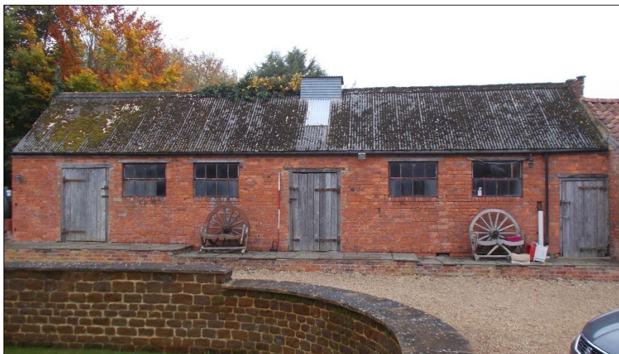
Fig 12: The west range, looking north. 2m scale rod.
