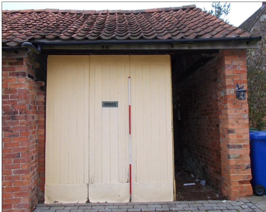
Fig 9: The eastern bay of the east range showing the sliding garage door, looking north. 2m scale rod.
