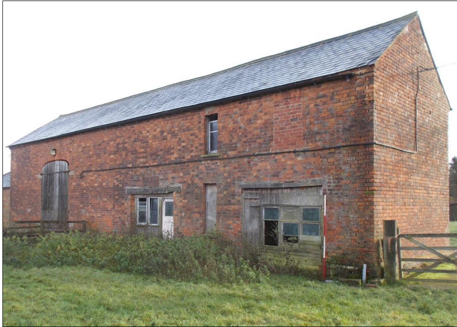
Fig 9: The west elevation, looking north-east. 2m scale rod.
