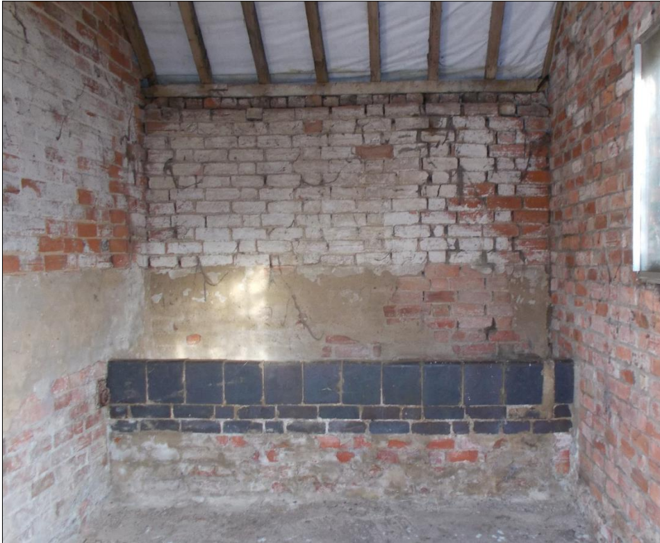
Fig 29: Room G10 showing the brick-built manger, looking north.
