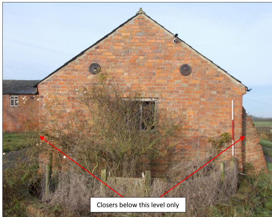
Fig 16: The eastern range, east gable wall, looking west. 2m scale rod.
