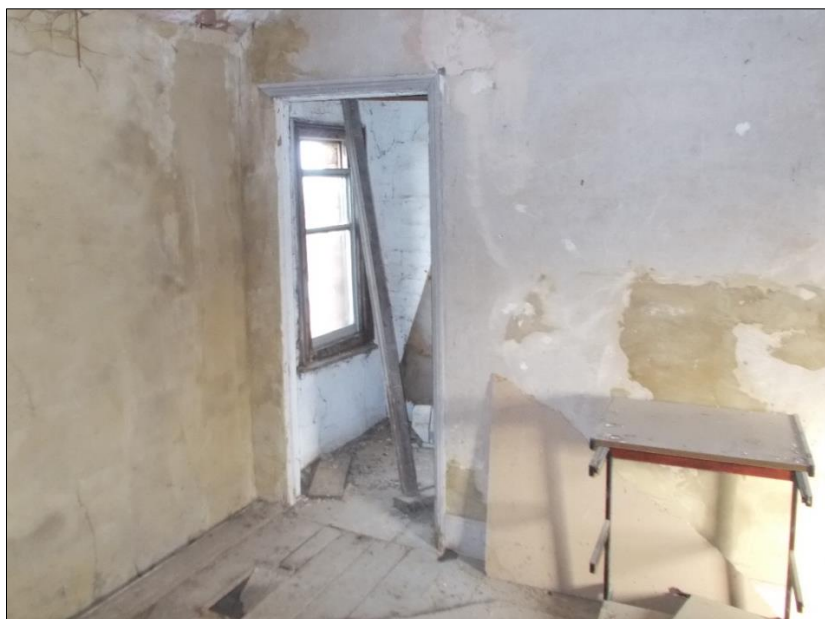
Fig 21: Room F2 looking north-west into the former top stairs landing.
