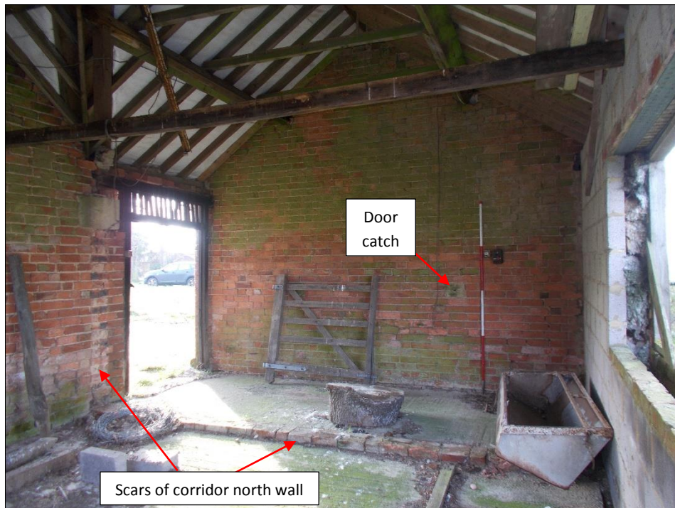
Fig 14: The corner room, looking south-east. Note scars of former corridor wall and breeze block re-build to right. 2m scale rod.
