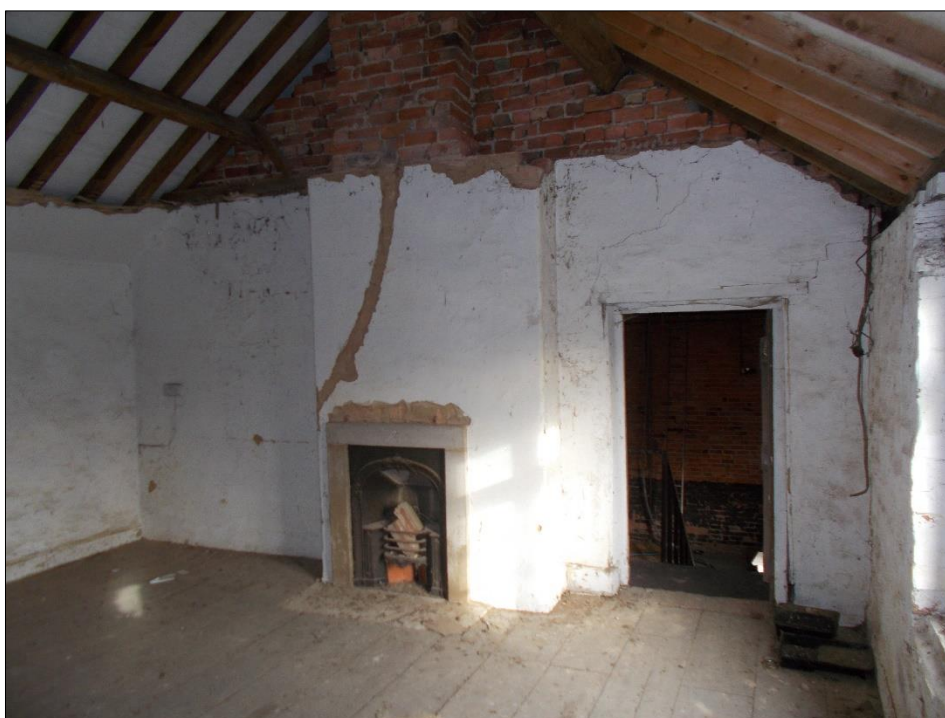
Fig 23: Room F3, showing original fireplace and grate and secondary doorway in the north wall.
