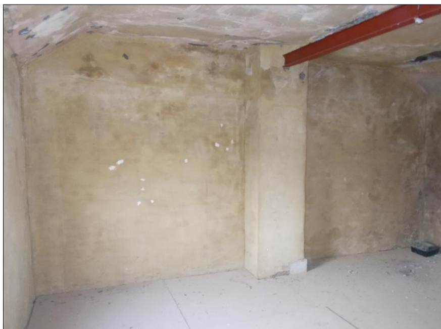
Fig 22: Room F2, looking south showing chimney stack from G1 below. Note modern RSJ.
