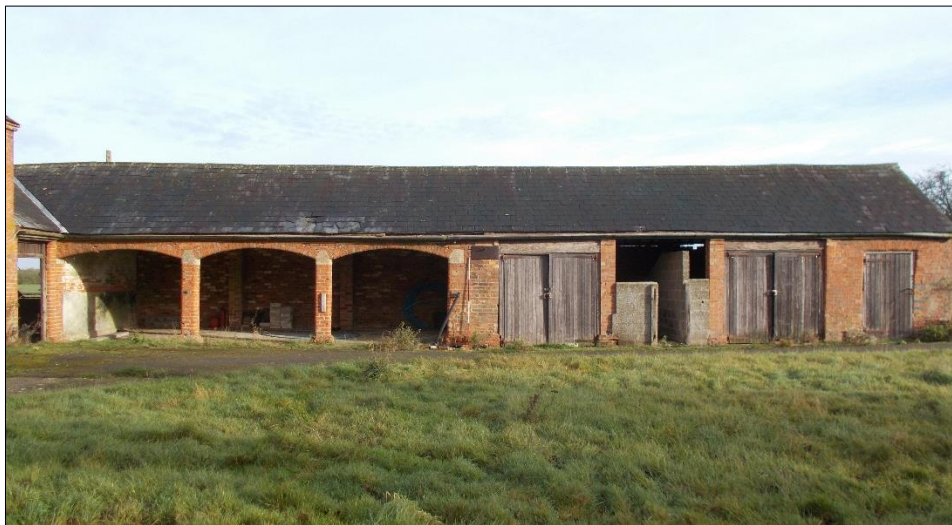
Fig 12: The south elevation of the eastern range, looking north. 2m scale rod.
