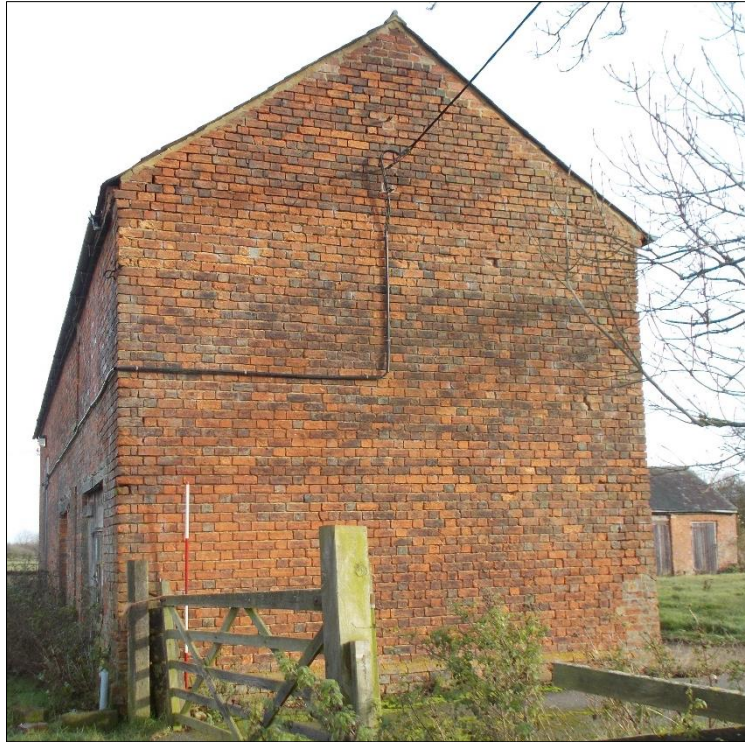
Fig 8: The south gable wall, looking north. 2m scale rod.
