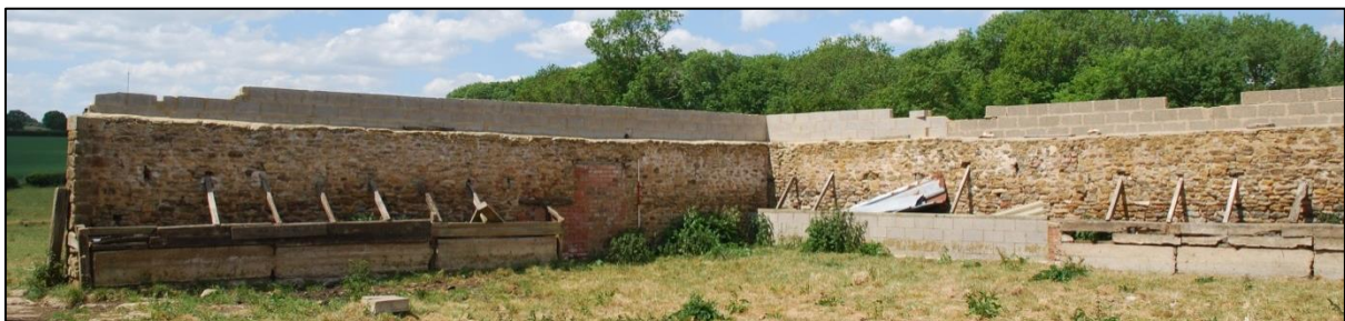
Fig 23: Vestiges of the missing west and south ranges. The uppermost blockwork and interior troughs were entirely related to the modern At-cost type shed; scale 2m
