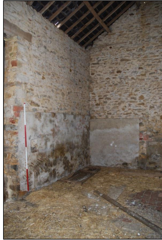
Fig 7: Barn interior with scars of shepherd's hut and lamp niche; scale 2m
