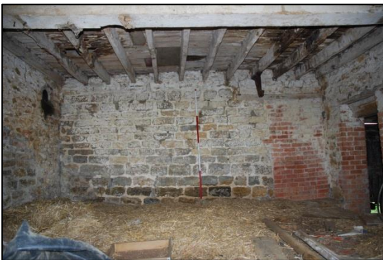
Fig 10: South wall of the corner room with bearing at left and hanging stirrup visible. Note blocked door and secondary doorway to the right. Scale 2m
