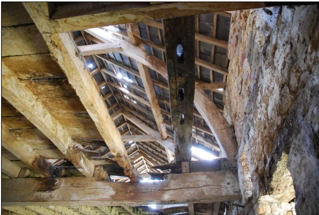
Fig 15: Looking south at the northernmost Cruck Truss, collar and sling-brace, through the redundant stair aperture. The morticed timber lies there loose by chance.
