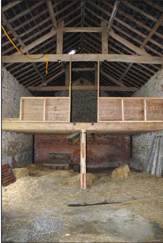
Fig 6: Barn interior with east end hayloft; scale 2m
