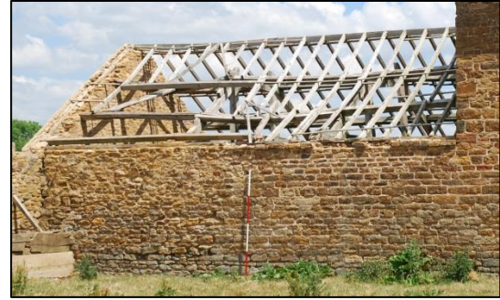
Fig 9: Rear (farmyard) face of cart hovel; Note the angled timbers of west range roof; scale 2m
