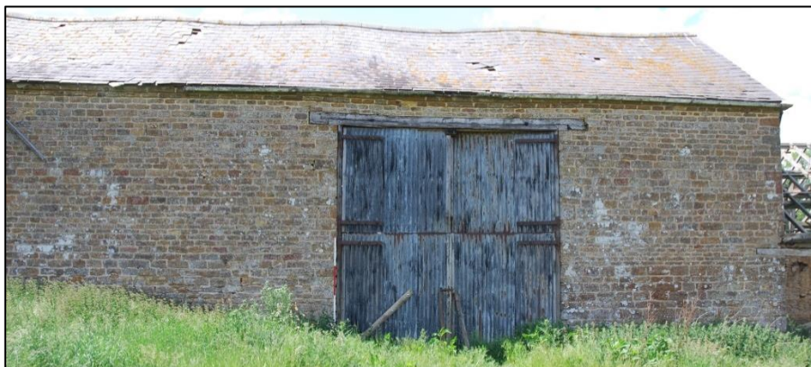
Fig 5: North side of the barn, looking south-west; scale 2m
