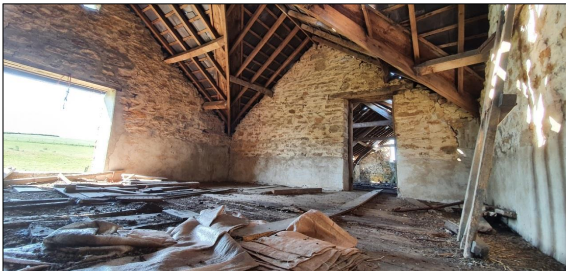
Fig 13: The first floor corner room connecting with the floor over the stable, looking south from the stairs. Note how the walls are plastered to about 70cm high. Unusually, the photo was taken from the stairs with extreme wide angle on a phone-camera for coverage and to avoid treading across the floor.
