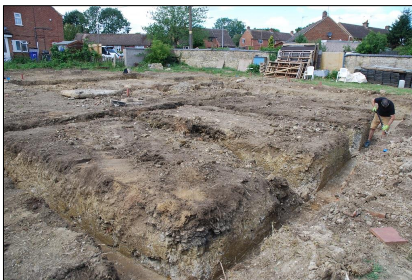
Fig 4: The site at the end of fieldwork, looking north-west. Extensive disturbance left many corners collapsing.
