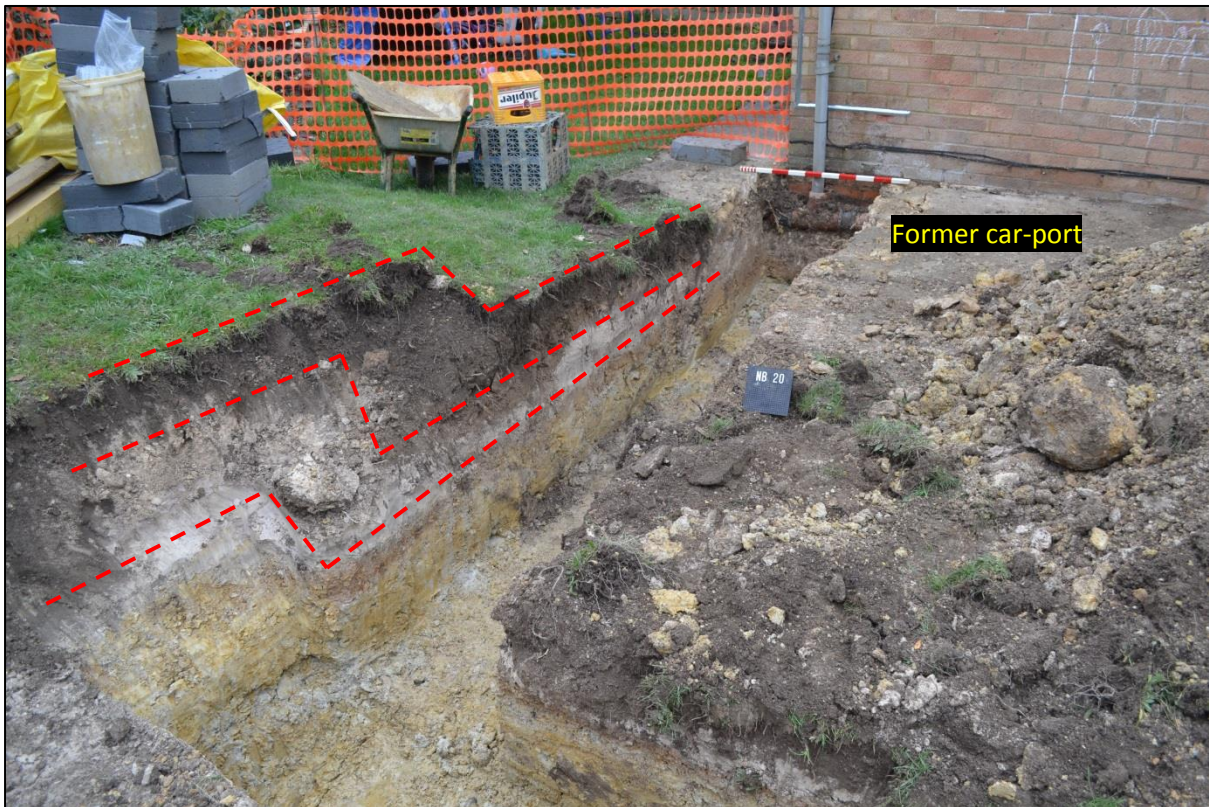
Fig 5: View of the northernmost foundation trench, showing the deliberate garden make-up above the terracing to the natural geology (dashed line). A slightly higher terrace lies to the west out of the picture at left as the plot narrows; Scale 1m
