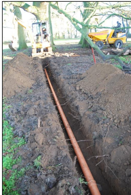
Fig 3: The outlet pipe trench, pipe inserted, looking north
