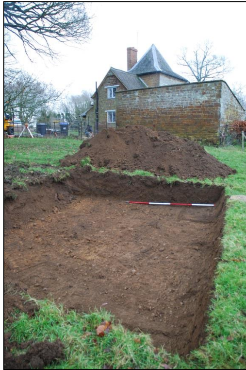
Fig 2: The soakaway, newly dug, looking towards Park Cottage; scale 2m
