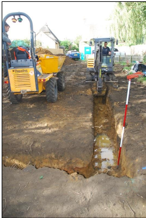
Fig 5: Machining the foundation trenches, looking west; scale 2m
