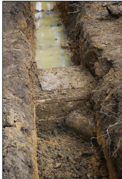
Fig 6: 8-inch ceramic collector drain and inspection chamber, looking east
