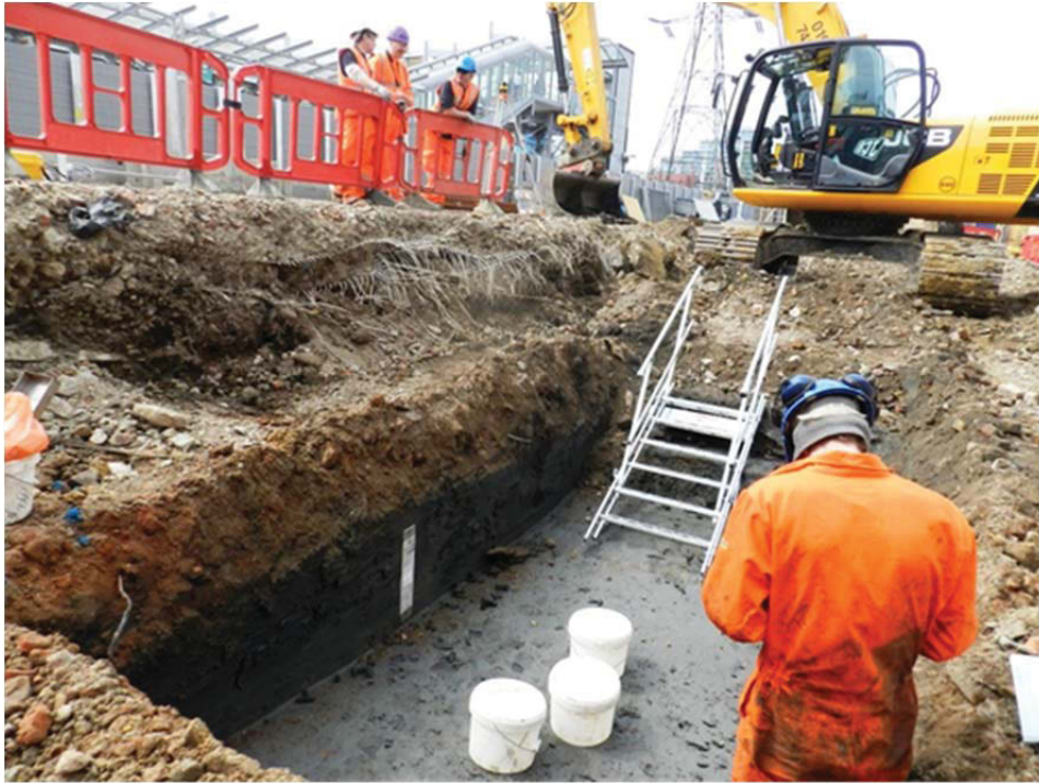
Photo 3 sampling the top of the trench, looking west
