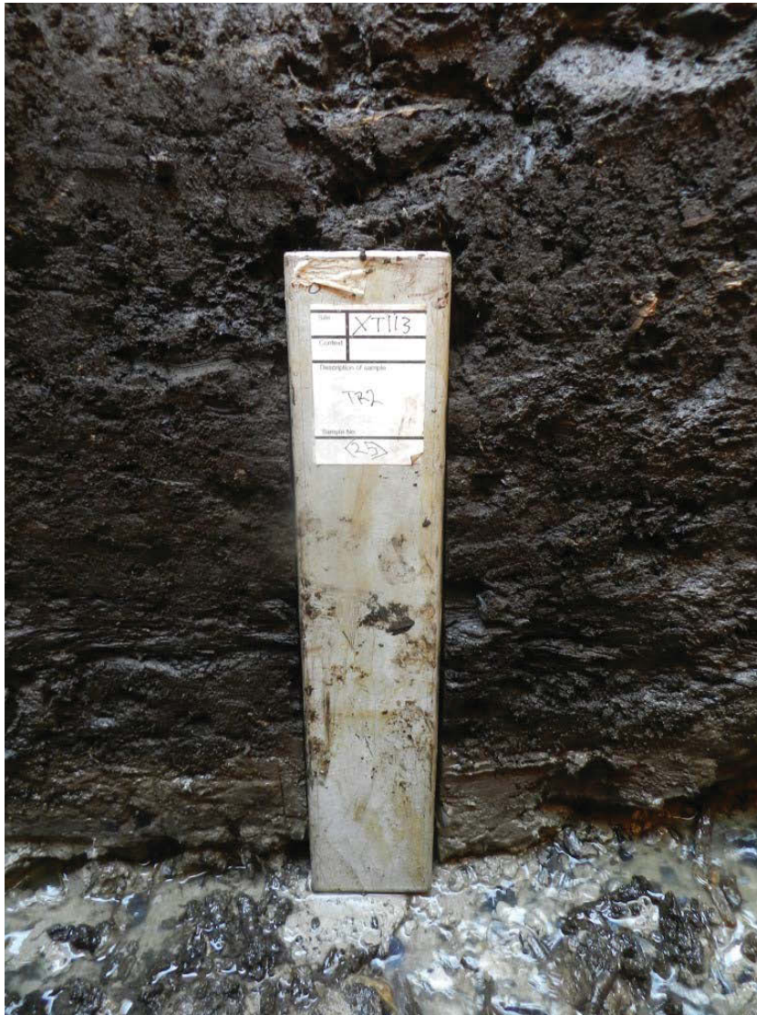
Photo 4 monolith <25> with water undermining the section
