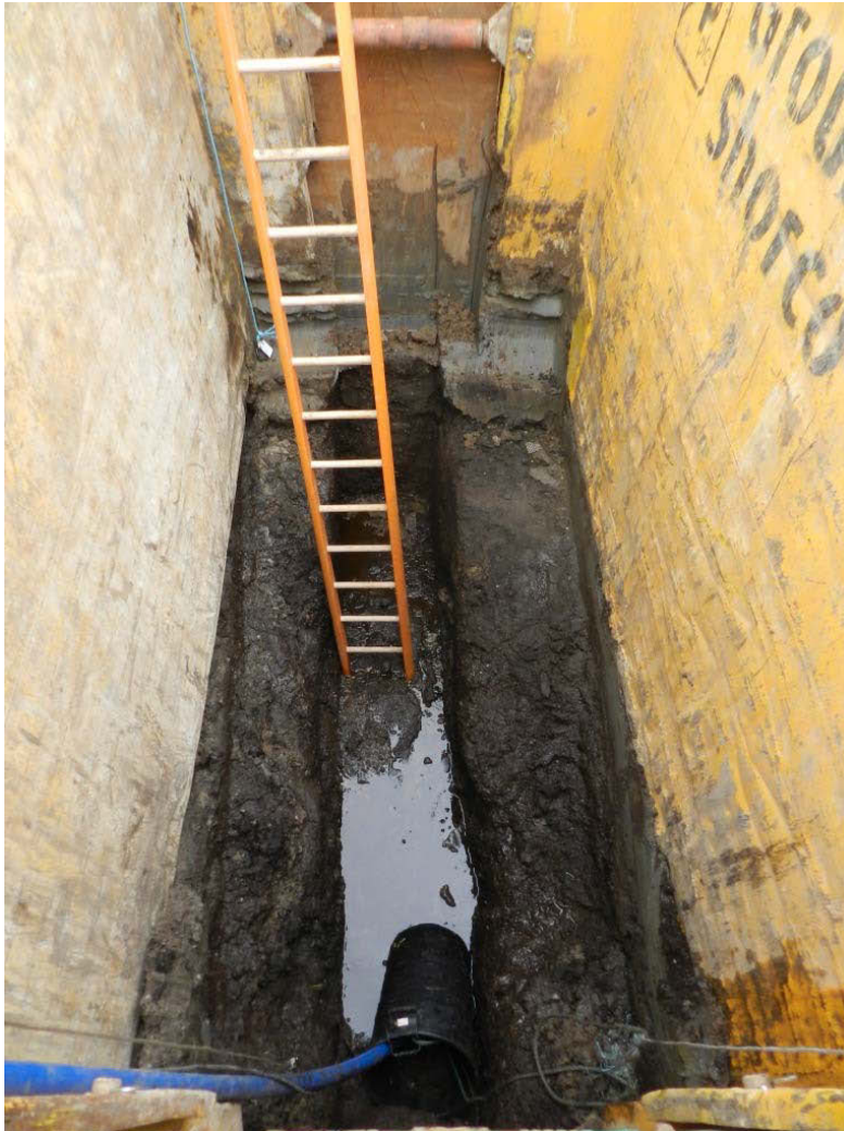
Trench 1: Looking north, wood peat exposed at base
