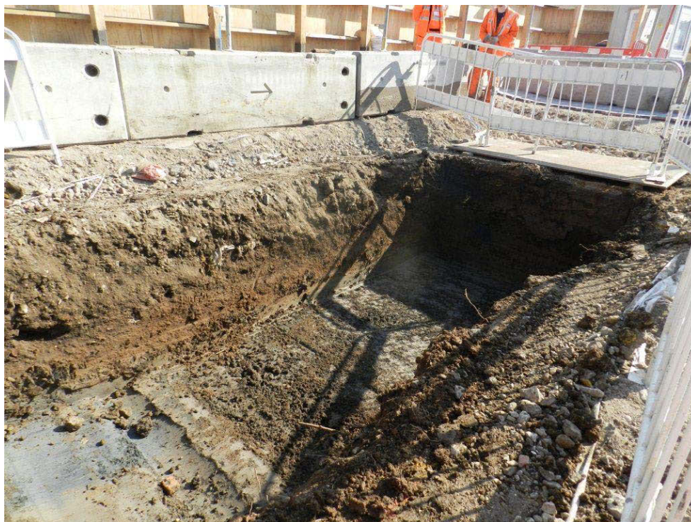
Trench 4: alluvium exposed beneath imported topsoil
