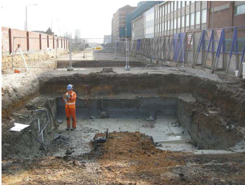
Photo 3 Looking east, sampling of upper alluvial deposits.
