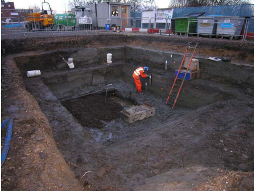
Photo 1, Trench 1, looking north-west, sampling of transition between upper clay and lower peats.
