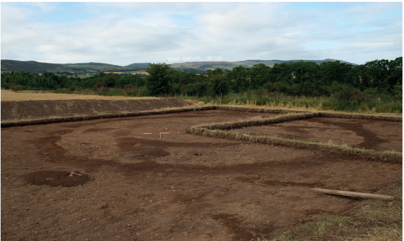
Figure 7.3 General view of excavations in Trench F with baulk still in place
