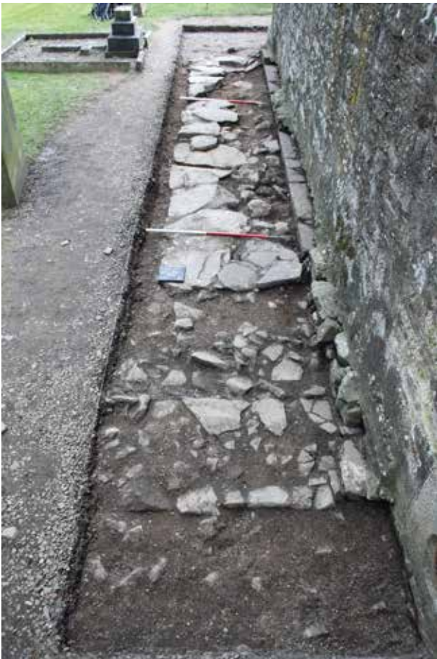
Figure 7.14 Foundations of Phase 4B Laird's Stairs
