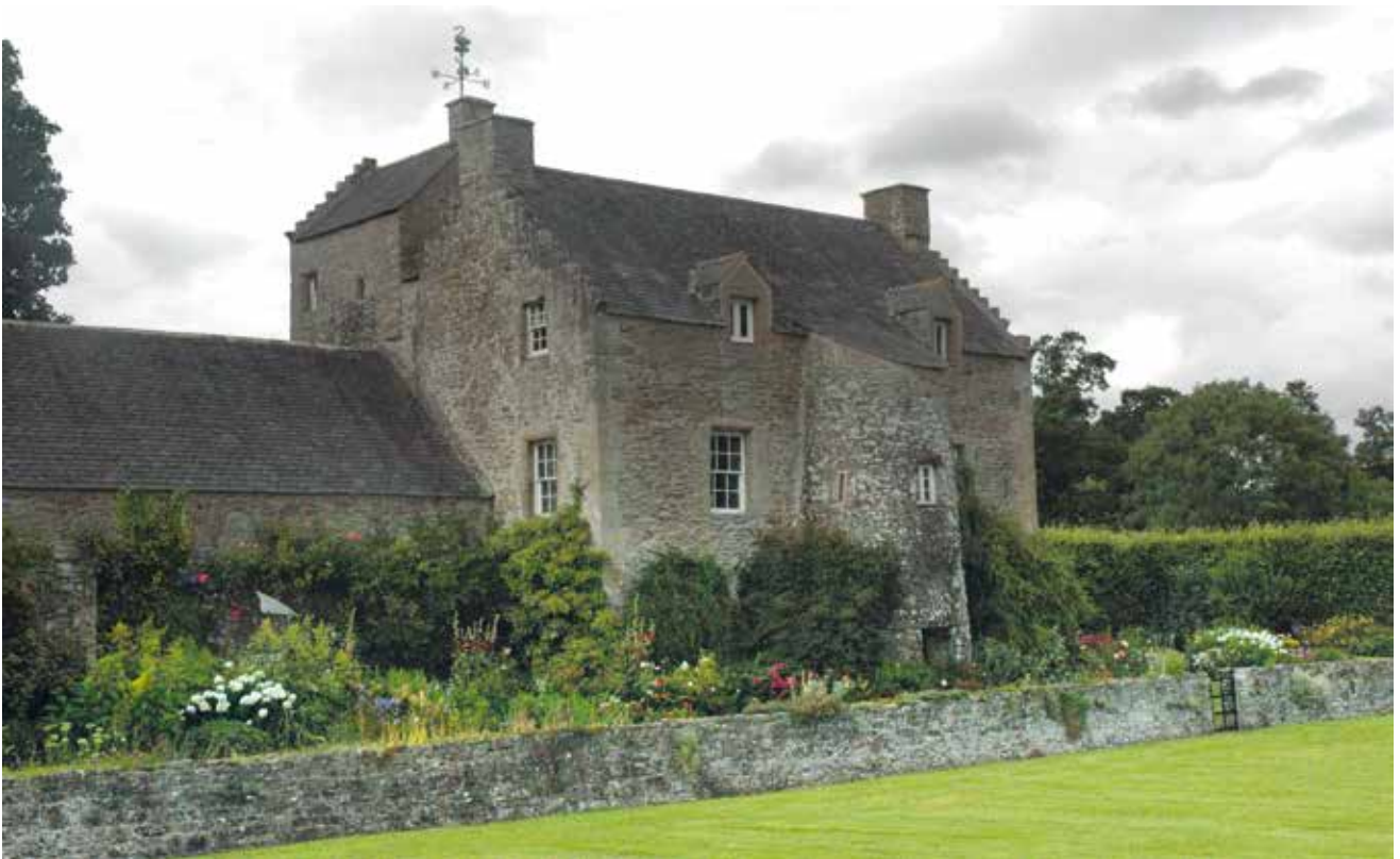
Figure 9.23 South elevation of Old Invermay House, with round stair tower probably added as part of remodelling in 1633
