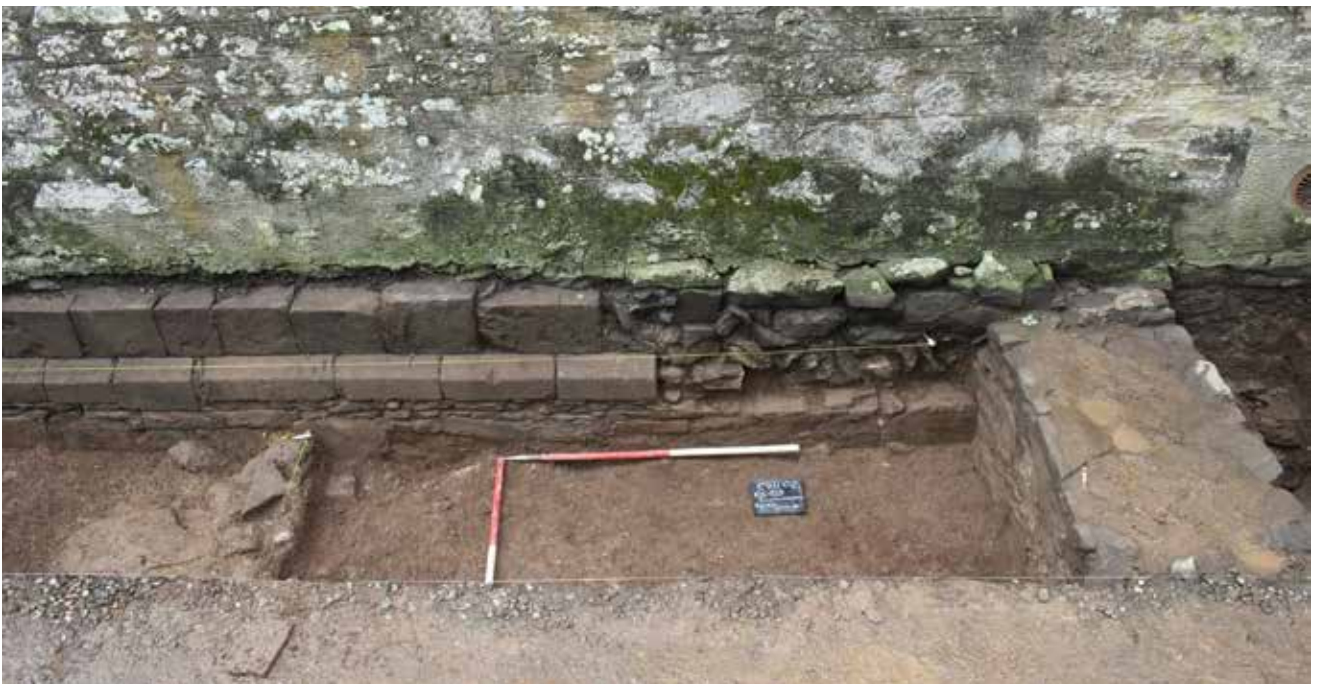
Figure 7.9 The walling around the blocked doorway
