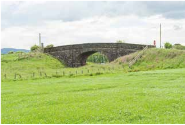
Figure 2.3 Viaduct over railway, leading to Milton of Forteviot
