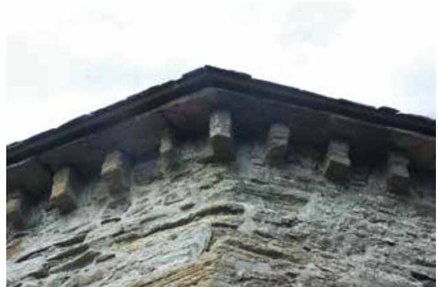
Figure 9.21 Detailed view of the Dovecot showing corbelled wall head
