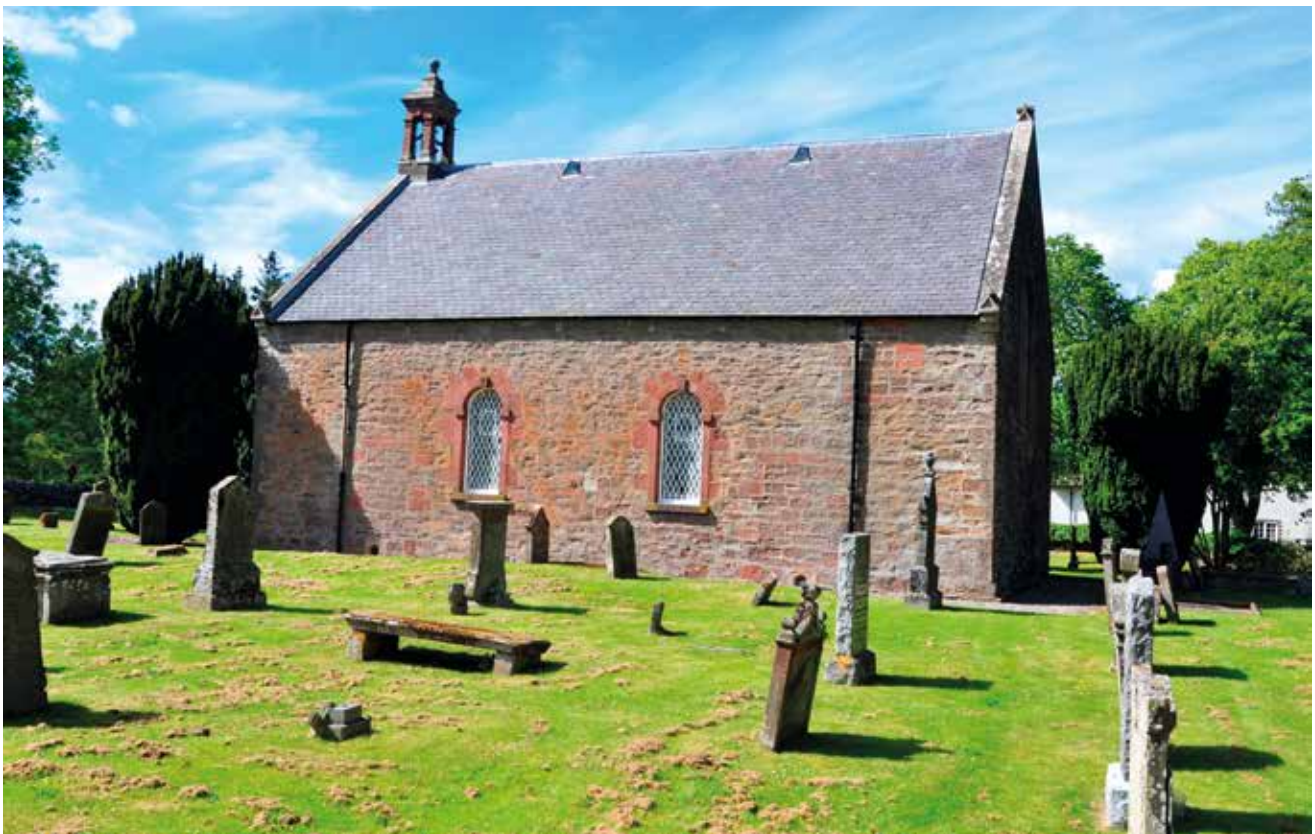
Figure 2.12 South elevation of Forteviot church showing blocked window and doorways of 1778 church
