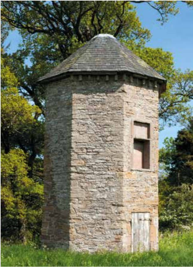
Figure 9.20 View of the Dovecot from the west. The ashlar quoins are of the same stone as the Old House of Invermay. The form of the recently restored roof may not reflect the original design
