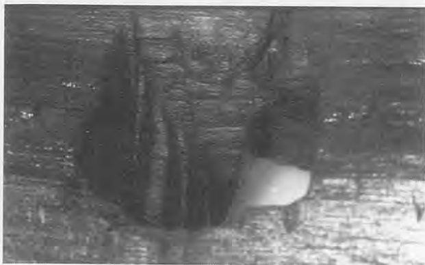
Fig 107 Toolmarks in plank mortise.
